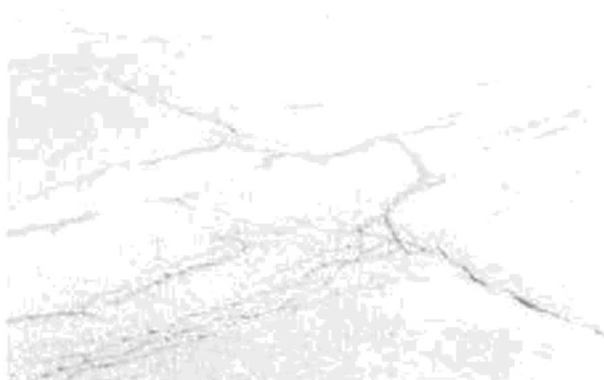
Figure 4. Extent of distress prior to paving.
