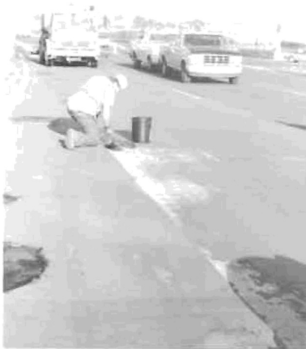
Figure 6. A cold-pour material was used to cover the area where the membrane was removed.
