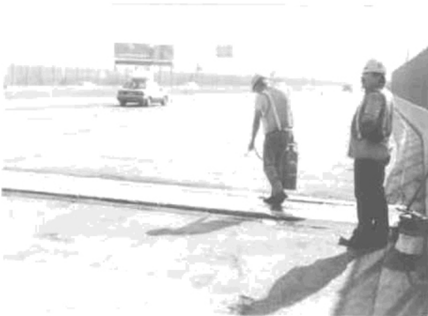
Figure 8. Preparing the joint prior to SMA placement.
