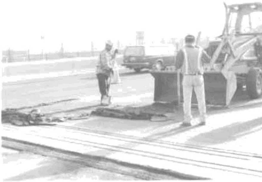
Figure 7. Removing the taper at the expansion joint.
