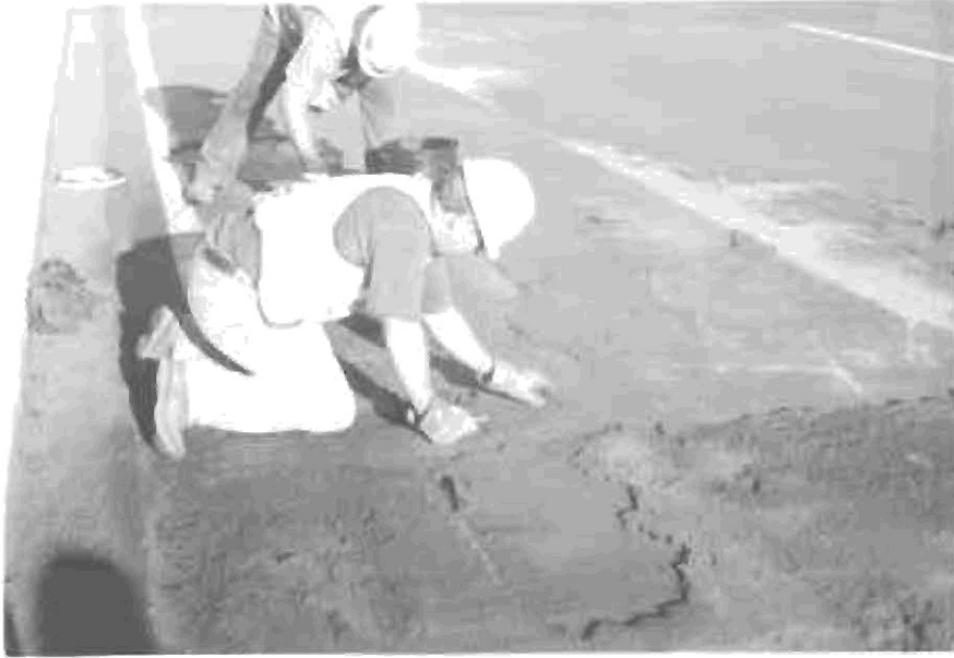
Figure 5. The exposed membrane was removed.
