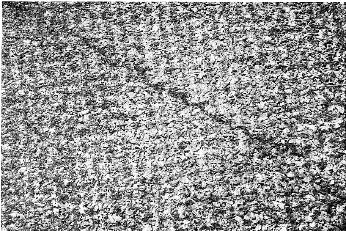
FIGURE 15. MINOR CRACKING IN LATEX RUBBER MODIFIED PFC RUNWAY AT OAKLAND PONTIAC AIRPORT
