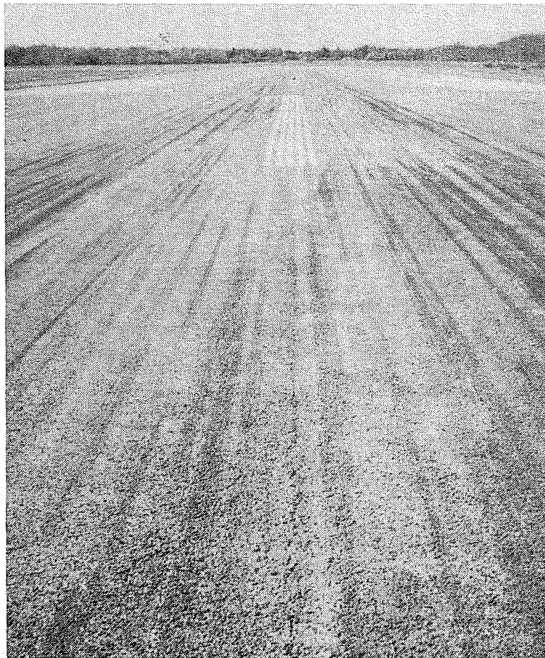
FIGURE 16. LATEX RUBBER MODIFIED PFC RUNWAY AT BISHOP INTERNATIONAL AIRPORT
