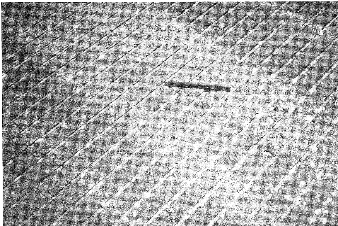
FIGURE 19. TRANSVERSE GROOVES CUT IN LATEX RUBBER MODIFIED RUNWAY PAVEMENT AT DETROIT CITY AIRPORT
