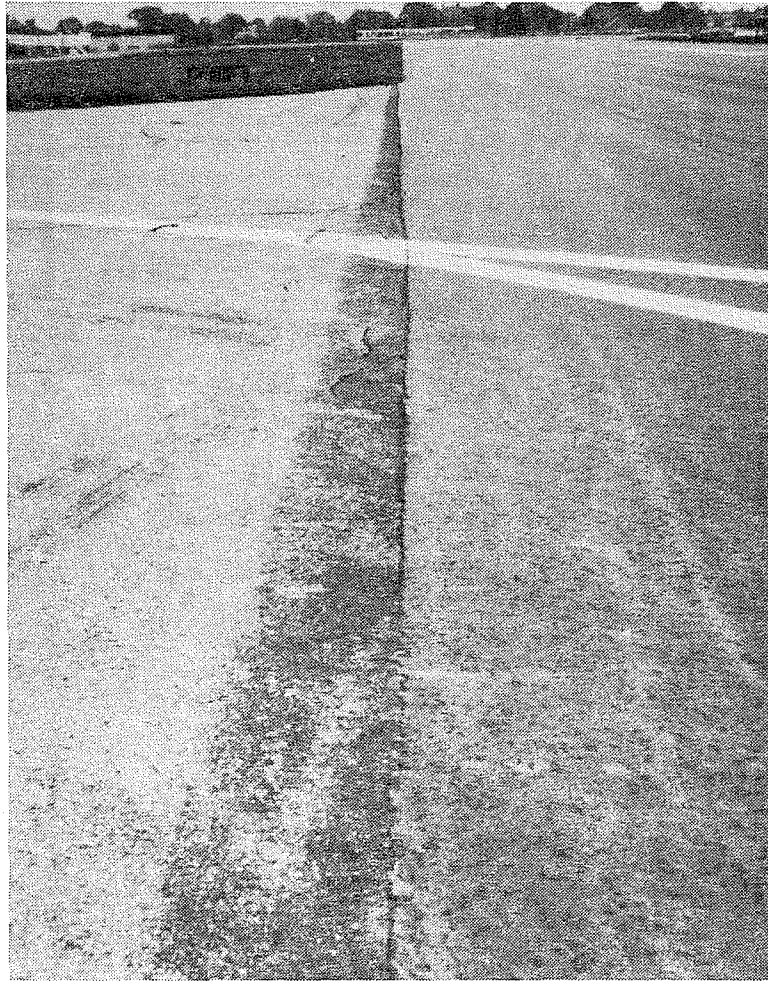
FIGURE 17. LATEX RUBBER MODIFIED RUNWAY (RIGHT) AT CAPITOL CITY AIRPORT
