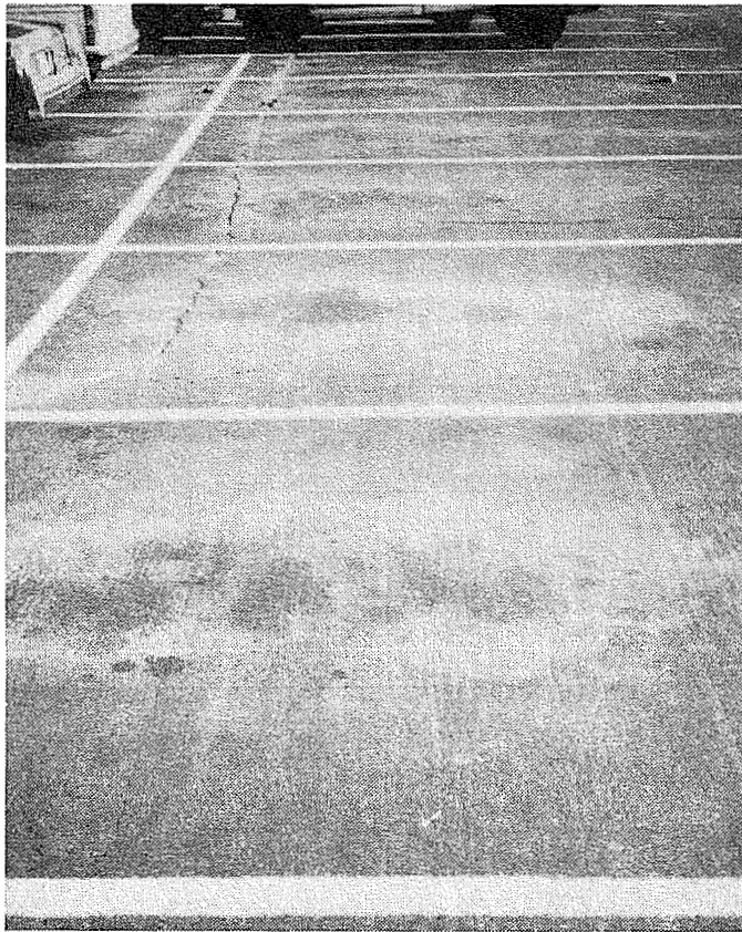
FIGURE 13. MODERATE LOSS OF FUEL-RESISTANT SEALER ON DFW PARKING LOT
