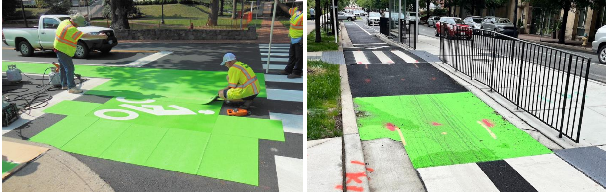
Figure 10. Thermoplastic and Methyl Methacrylate Green-Colored Pavement Markings: (left) preformed thermoplastic; (right) methyl methacrylate
