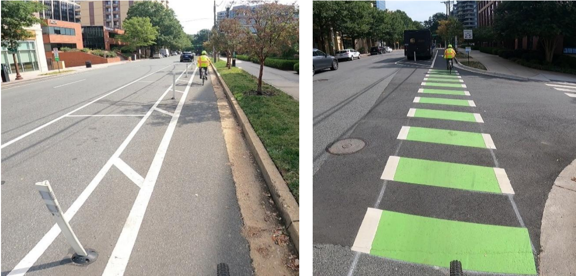
Figure 29. Clarendon Boulevard Bicycle Lane: (left) flexpost-separated bike lane from North Quinn Street to North Queen Street; (right) thermoplastic skips at Clarendon Boulevard and North Queen Street intersection
