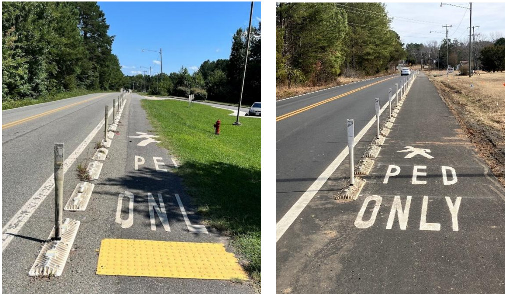
Figure 22. Sinai Road Pedestrian Lane in Halifax County: (left) vegetation overgrowth on shoulder in August 2025; (right, courtesy of Roy Sage) after repaving and reinstallation in January 2026
