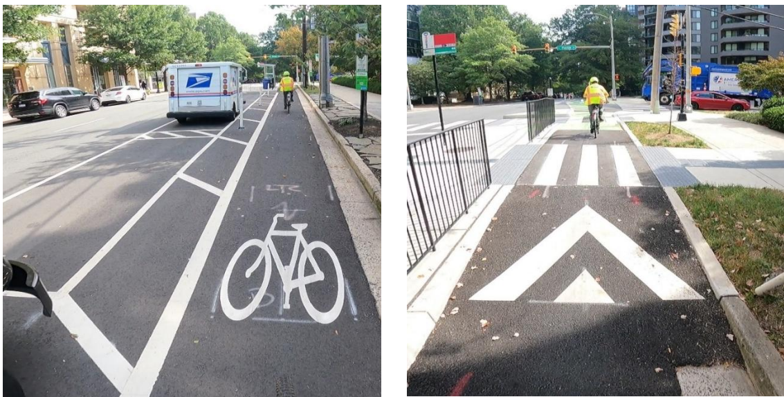
Figure 30. Clarendon Boulevard Bicycle Lane: (left) flexpost-separated bike lane from North Queen Street to North Pierce Street with missing flexposts; (right) crosswalk to bus boarding island slightly west of North Pierce Street intersection
