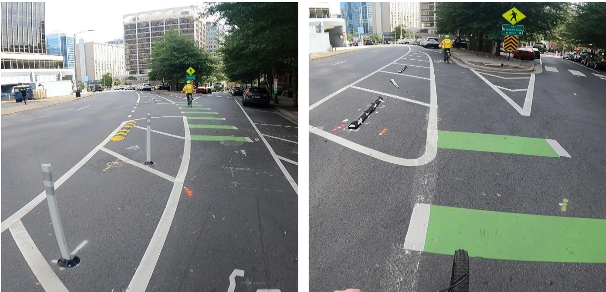
Figure 34. Clarendon Boulevard and 17th Street North Intersection: (left) flexposts and thermoplastic green-colored pavement marking skips; (right) downed flexpost
