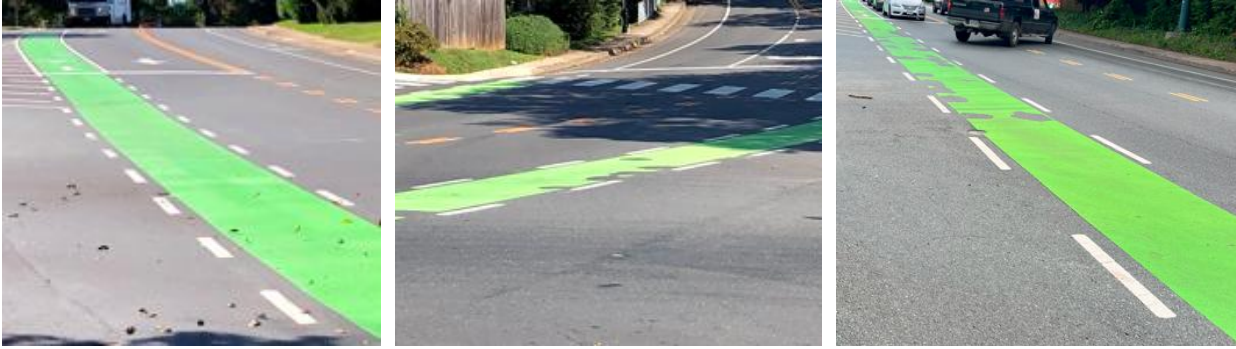
Figure 12. A Site in Charlottesville with Solid Green Thermoplastic: (left) shortly after installation; (center) from the opposite angle, wear after 1 year; (right) additional wear after 5 years
