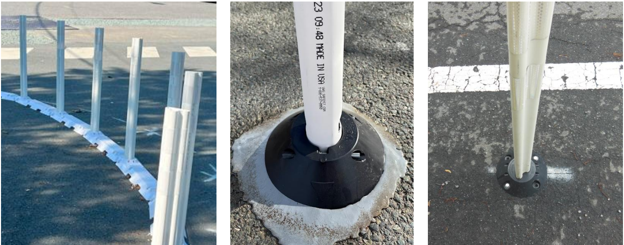
Figure 14. Examples of Flexpost Installations: (left) on a curb base; (center) individually mounted using epoxy; (right) individually mounted using two of four bolt holes
