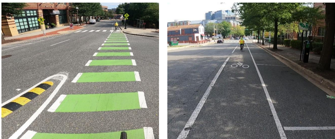
Figure 26. Clarendon Boulevard Unprotected Bicycle Lane: (left) thermoplastic skips at Clarendon Boulevard and North Scott Street; (right) standard bicycle lane from North Scott Street to North Rhodes Street
