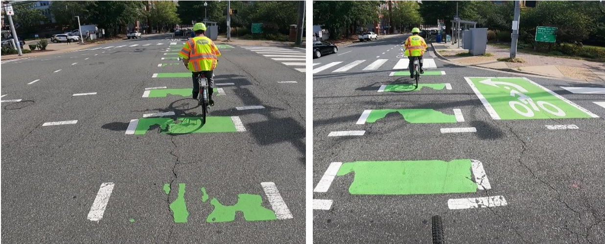
Figure 27. Clarendon Boulevard and North Rhodes Street: (left) thermoplastic skips; (right) two-stage turn box
