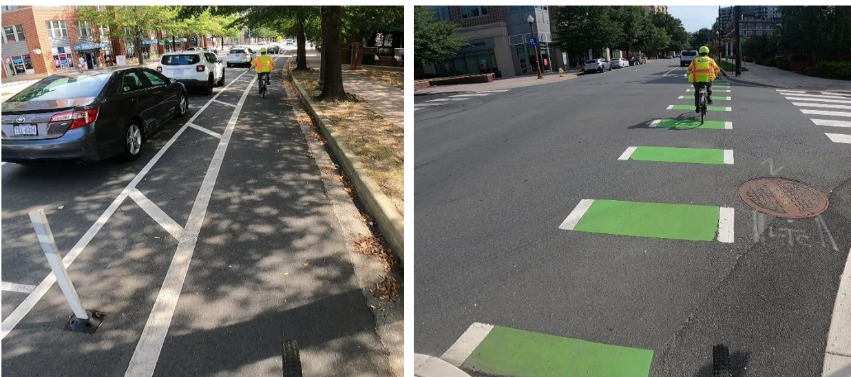
Figure 28. Clarendon Boulevard Bicycle Lane: (left) flexpost-separated bike lane from North Rhodes Street to North Quinn Street with missing flexposts; (right) thermoplastic skips at Clarendon Boulevard and North Quinn Street intersection
