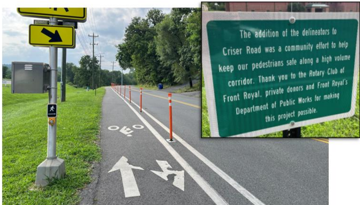
Figure 19. West Criser Road Bicycle and Pedestrian Lane Separated with Flexposts
