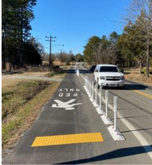
Figure 5. Flexposts Used for a Pedestrian Lane Along Sinai Road in Halifax County
