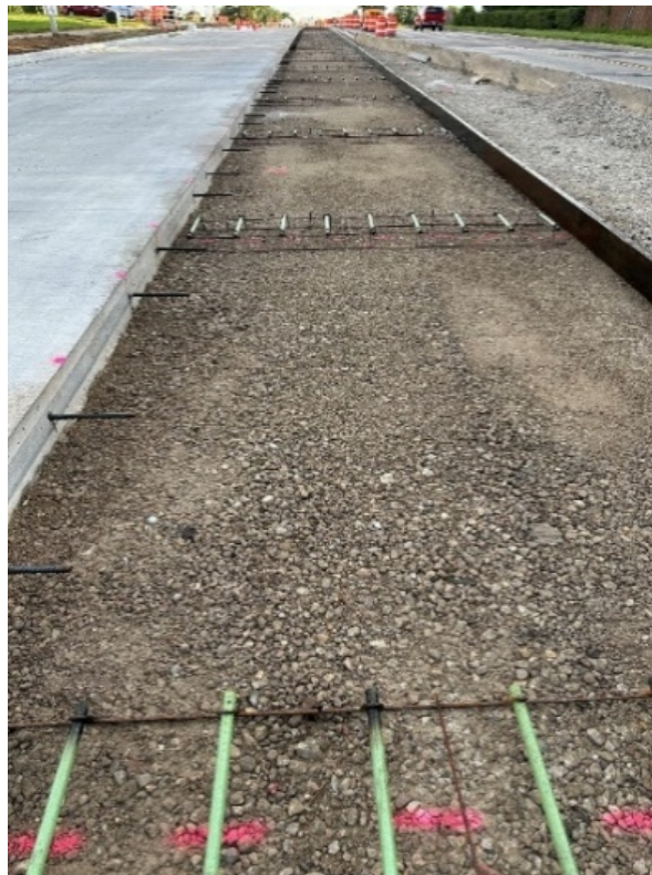
Figure 62. Image. Dowel bars ready for concrete pour.
