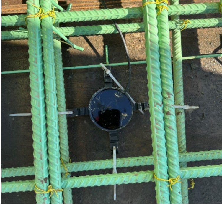
Figure 45. Image. Sensor secured to the bottom reinforcement with zip ties.
