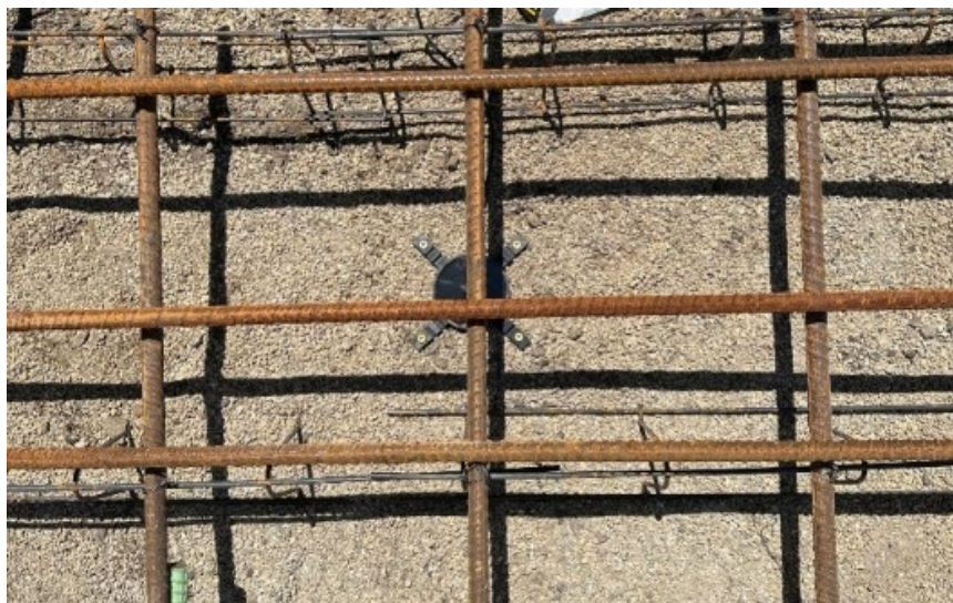
Figure 55. Image. Sensor 2 under the rebar.
