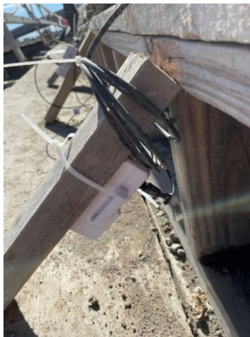
Figure 49. Image. Repositioned data loggers.
