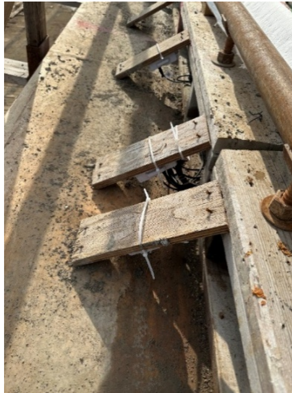
Figure 52. Image. Data loggers zip-tied to formwork supports.
