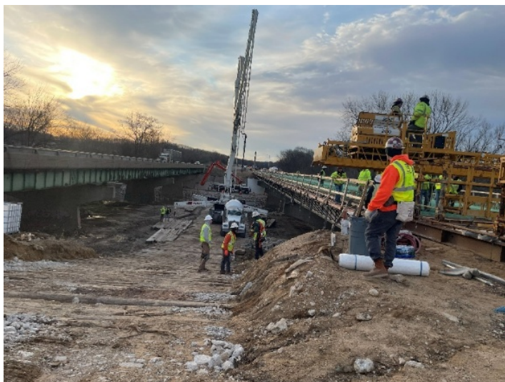
Figure 53. Image. Concrete truck down the slope to pump concrete to the bridge deck.
