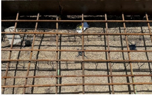
Figure 56. Image. Sensors nailed in place.
