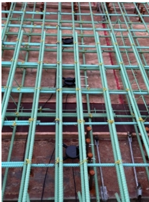
Figure 50. Image. Sensors zip-tied to rebar.
