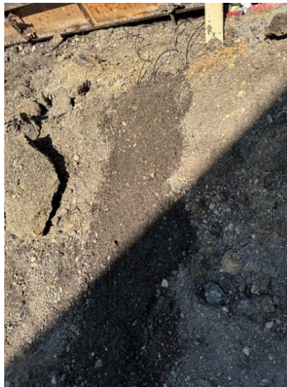
Figure 57. Image. Sensor cords buried outside of the formwork.
