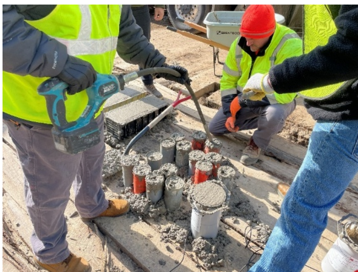
Figure 54. Image. Compacting the test specimens with a concrete vibrator.
