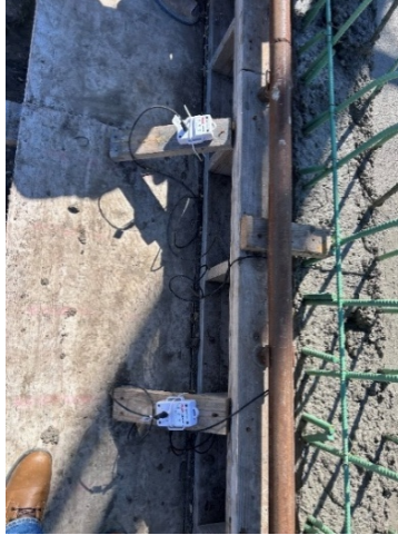
Figure 47. Image. Data loggers zip-tied to outside of formwork.
