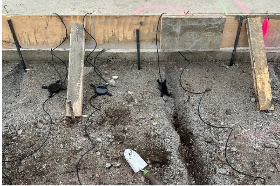
Figure 41. Photo. Trench for sensor cables.
