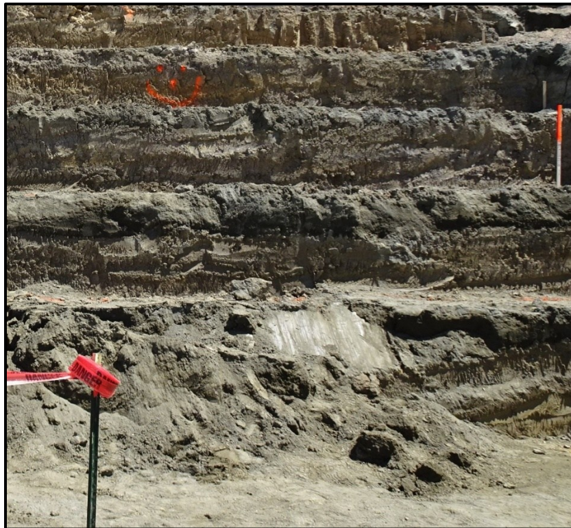
Figure 24. US 36 MP 50.05 Location of Slickensides Donating Failure Plane in Excavation.
