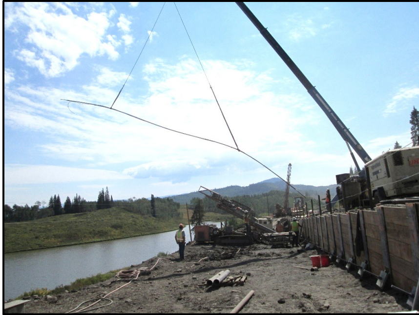
Figure 5. US 40 MP 156.7 depiction of installation of a tieback into the soldier pile lagging wall.
