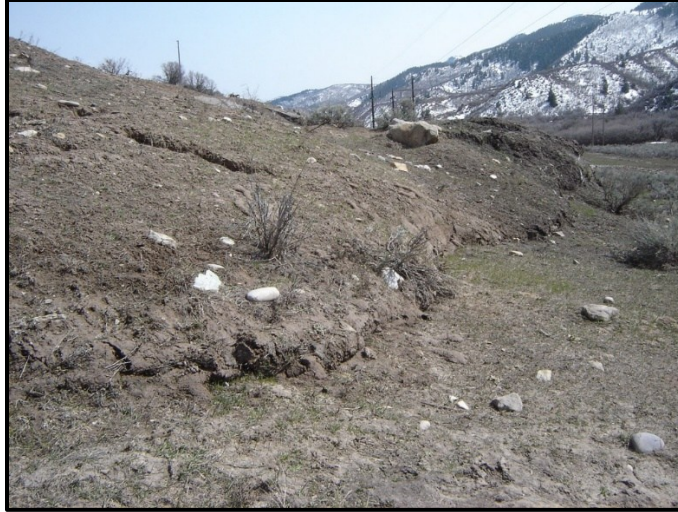
Figure 6. CO 13 MP 15.9 depicts toe of slope which failed as a bearing/slide and over-rode materials.
