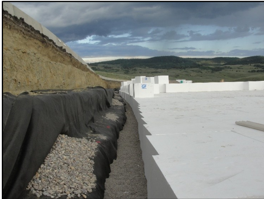
Figure 15. US 50 MP 108 depiction of construction of geofabric mitigation stabilization.
