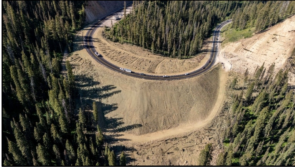
Figure 20. WY 22 MP 12.8 aerial view of embankment stabilization in 2025.
