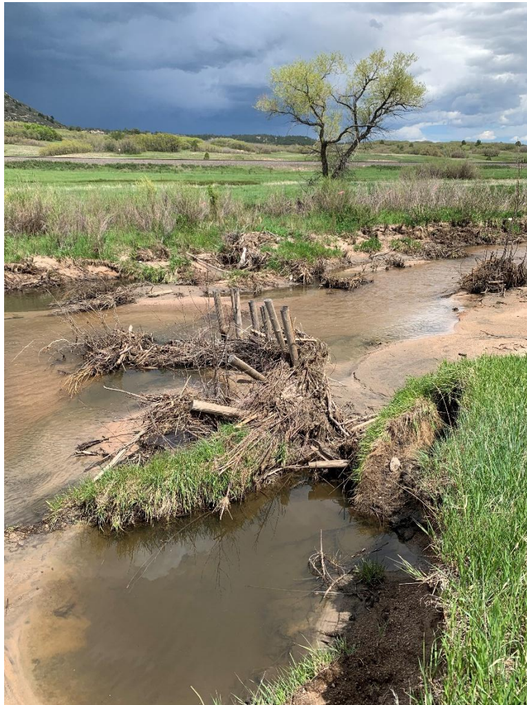
Figure 15. Post-flooding impacts at a beaver dam analog along East Plum Creek, Douglas County
