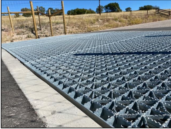
Figure 41. Surface of the wildlife guards in the I-25 South Gap Project.
