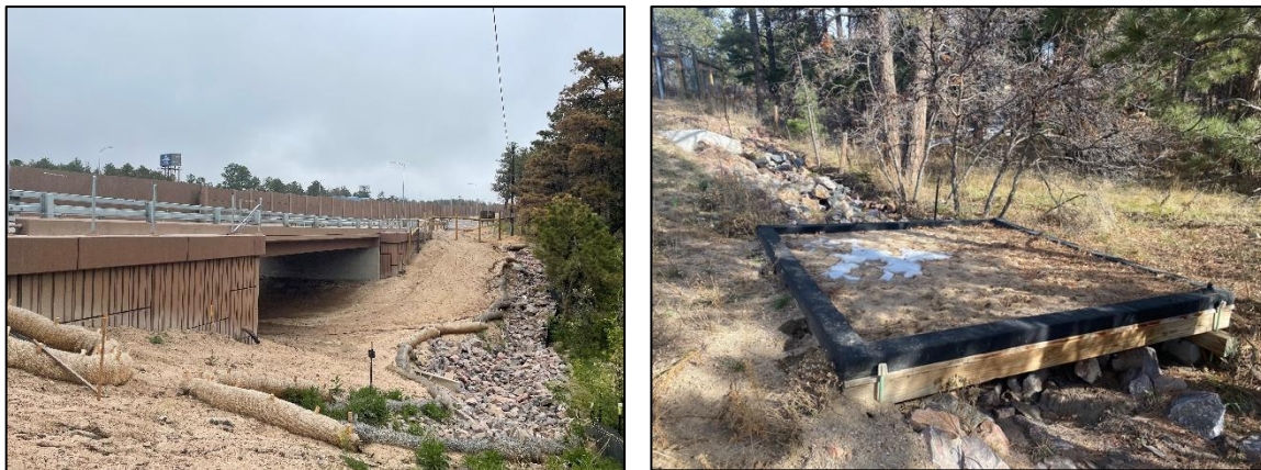
Figure 2. Riprap drainage running across the east entrance to the Monument Hill Underpass (left) and the natural surface 'deer bridge' installed over the riprap drainage to facilitate wildlife passage (right).
