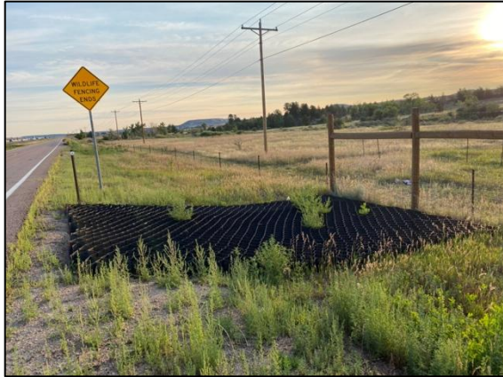
Figure 7. North fence end Geocell treatment along the east frontage road.
