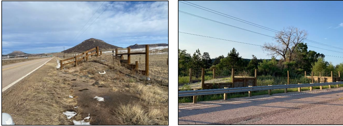
Figure 6. Example of one-sided escape ramp (left) and two-sided escape ramp (right).
