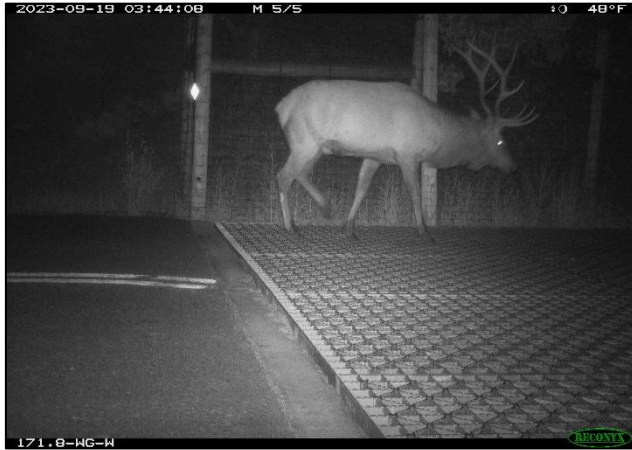
Figure 39. Bull elk successfully breaching the Upper Lake Gulch Road - West Wildlife Guard.
