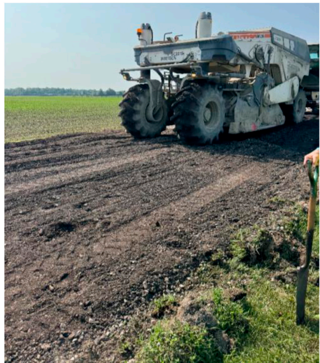
Figure 4.1 CIR Recycling Operations at SR 13 Project Site.
