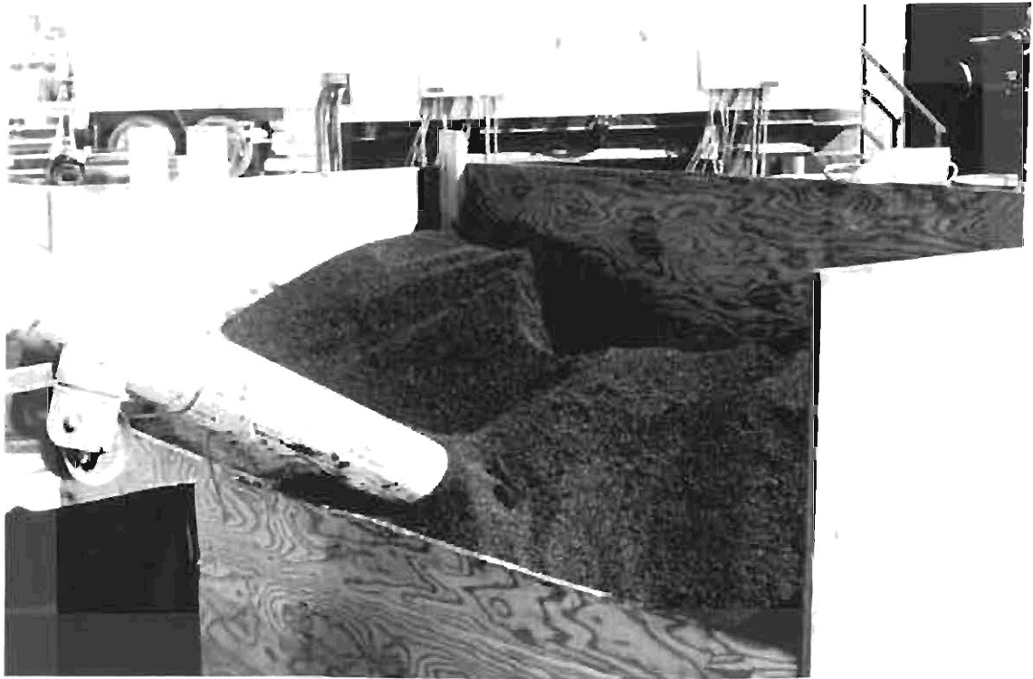
Figure 6. An auger was used to transport the crumb rubber to the RAP collar
