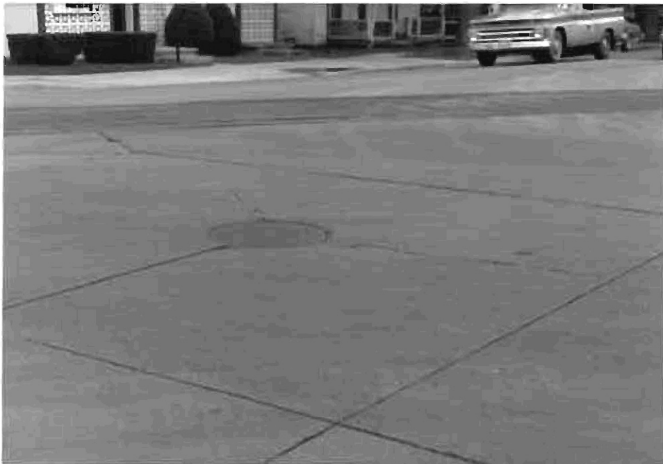
Photo 4: Formation of diagonal cracks due to presence of manhole and/or irregular joint spacing.
