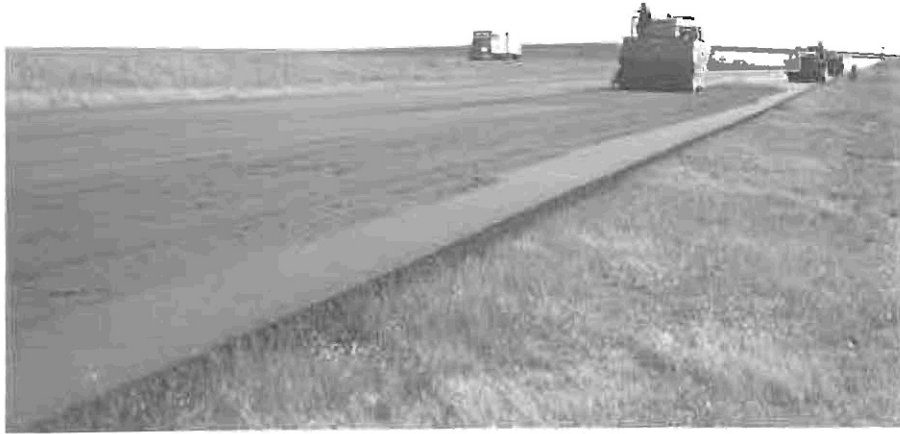
Figure 19. Pneumatic tire rollers tend to pick up the mat. This photo shows an extreme case.
