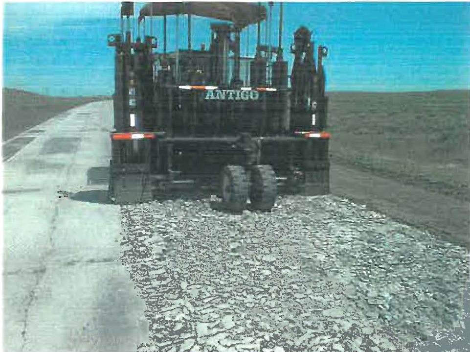
Figure 11. Multi-head hammer in action.
