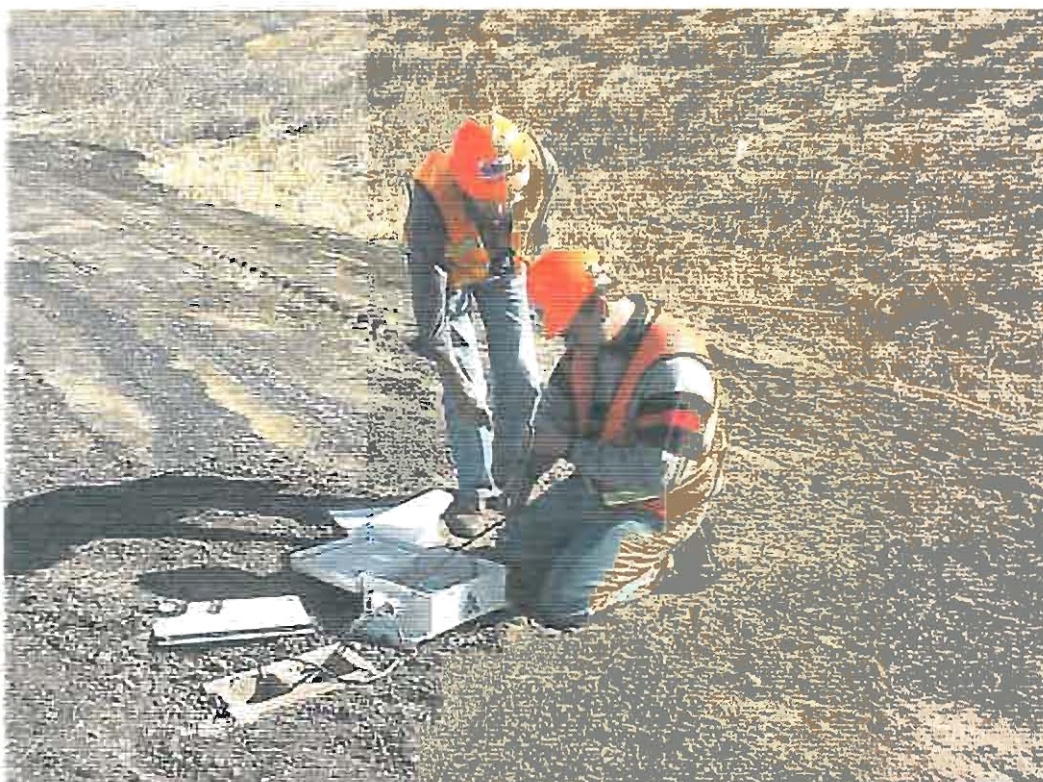
Figure 18. Installation of the moisture sensors.
