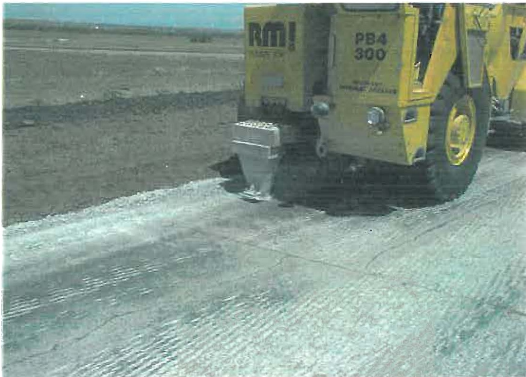
Figure 10. Resonant breaker in action.
