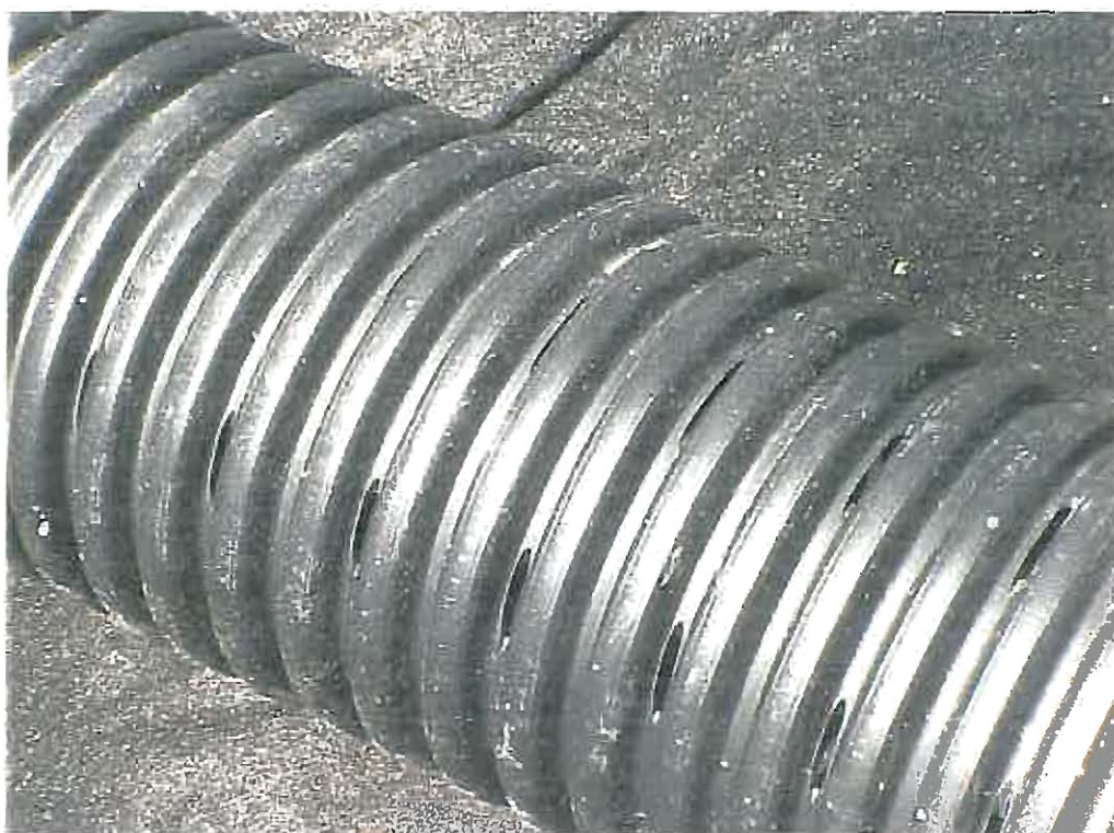
Figure 15. Close-up of perforated drainpipe & geotextile.
