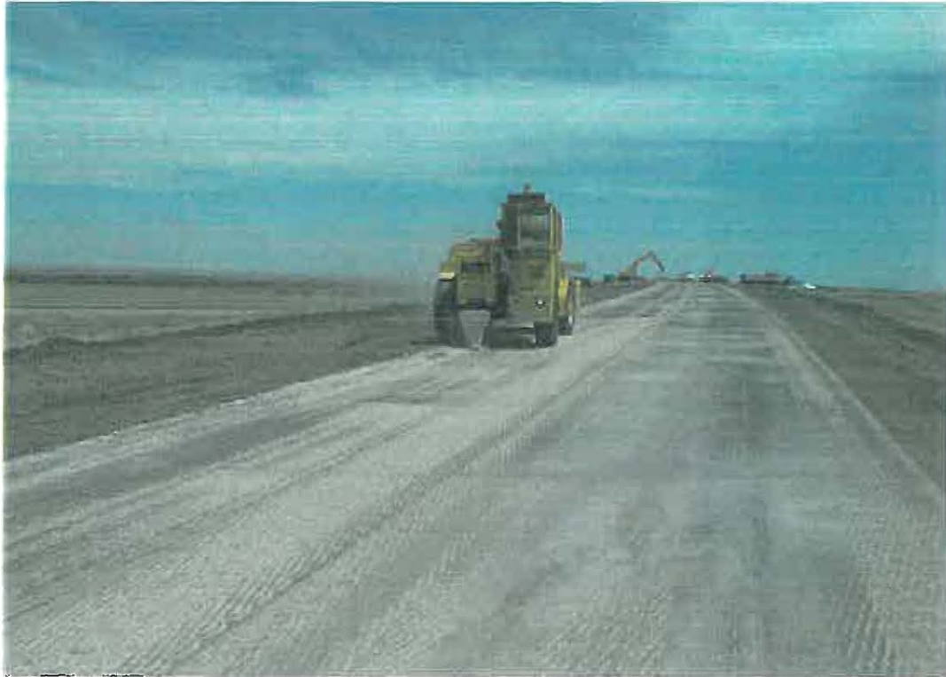
Figure 9. Resonant treatment process.
