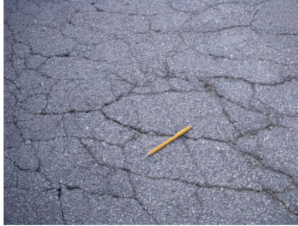
Figure A-11. Fatigue Cracking
