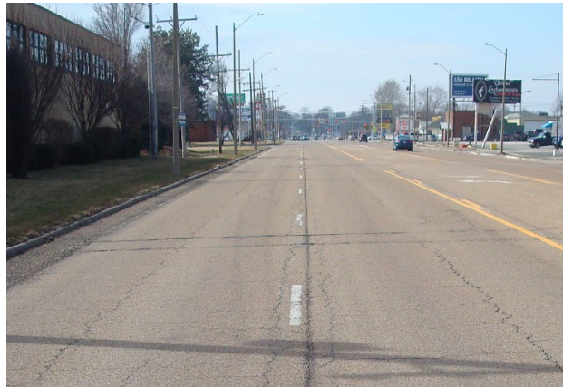
Figure A-10. Reflective Cracking
