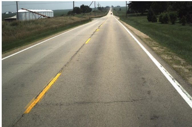
Figure A-8. Thermal Cracking
