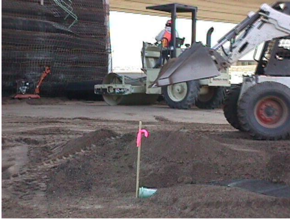
Figure B-25. The pipe used with the drainage blanket placed behind the reinforced backfill.
