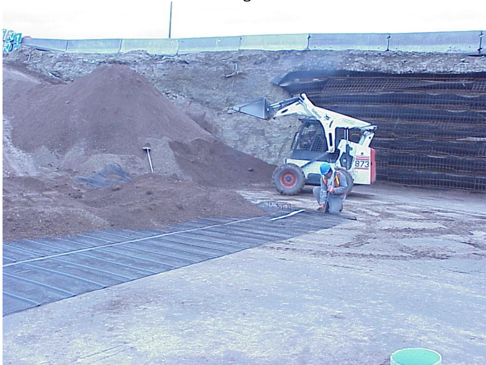
Figure B-20. The geogrid was connected at the wall end, rolled out, and then stretched by hand. The back end was staked to prevent geogrid movement while the fill was placed using a small loader. In the background is the steel reinforcement used to temporarily support the northern face of the Phase I structure.
