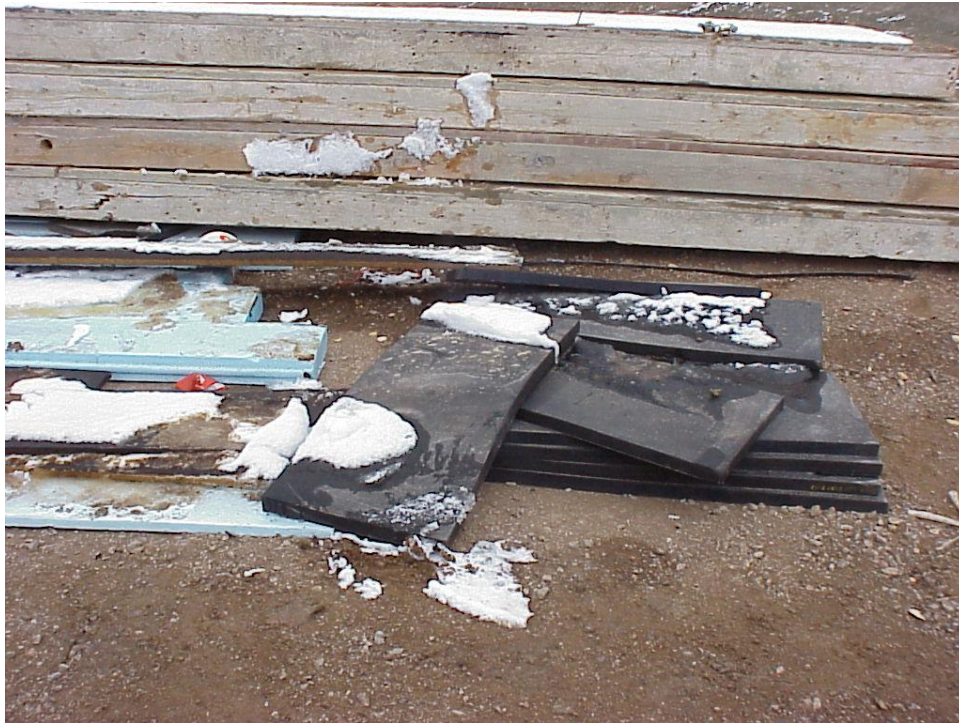
Figure B-30. These elastomeric bearing pads were installed on the abutment wall where the bridge girders are seated.
