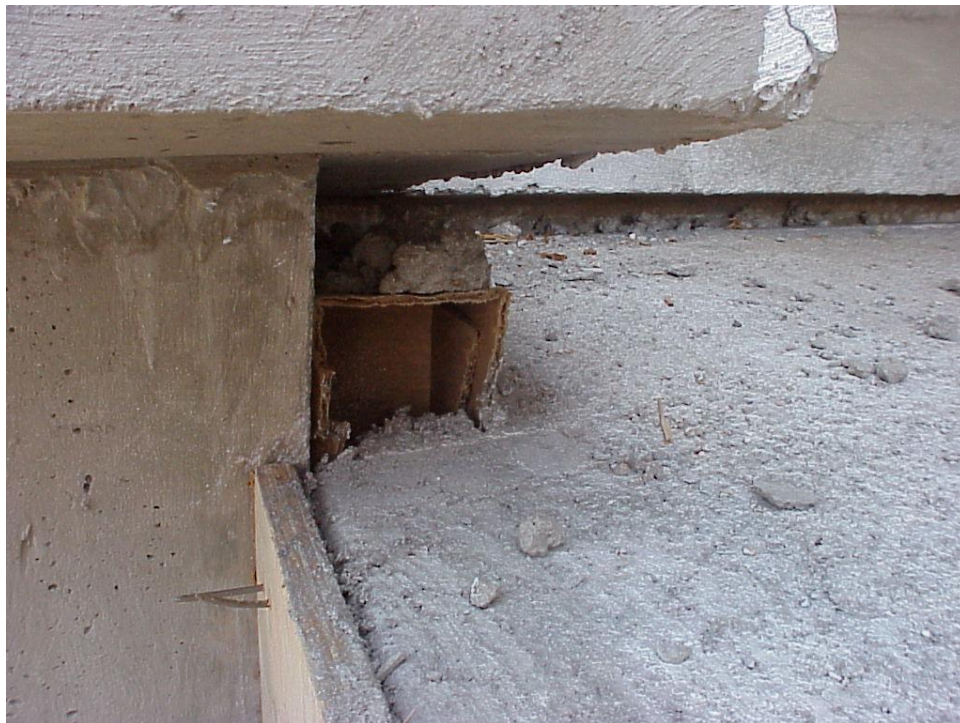
Figure B-40. Collapsible cardboard was placed in front of the bottom portion of the abutment wall behind slope paving (see figures 29 and 35).
