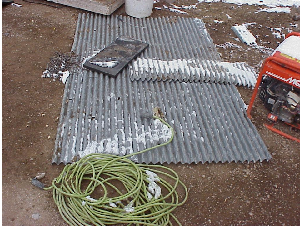
Figure B-39. This panel was used to give texture to the outside of surface of the concrete wing wall.
