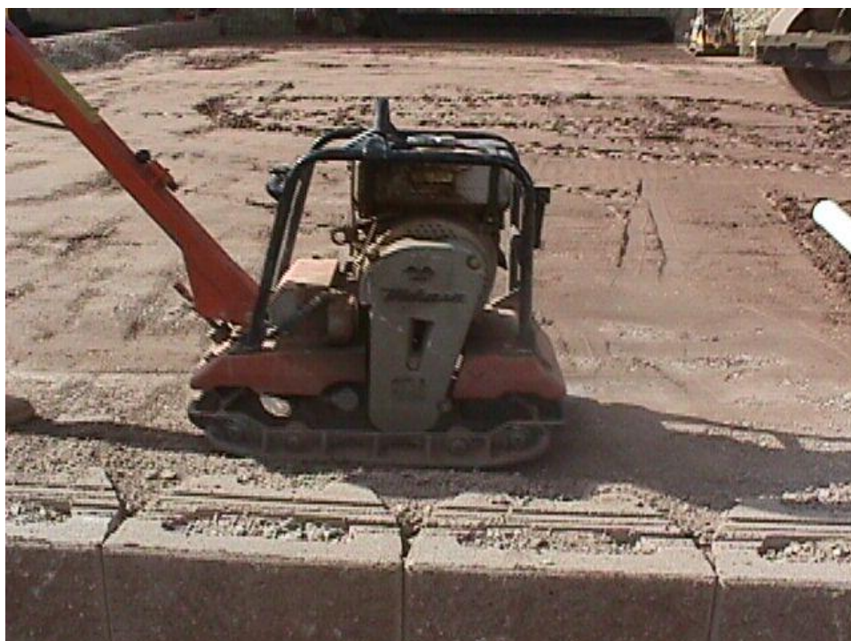
Figure B-22. Near the block facing, a small walk-behind compactor was used to prevent pushing the blocks out of position.
