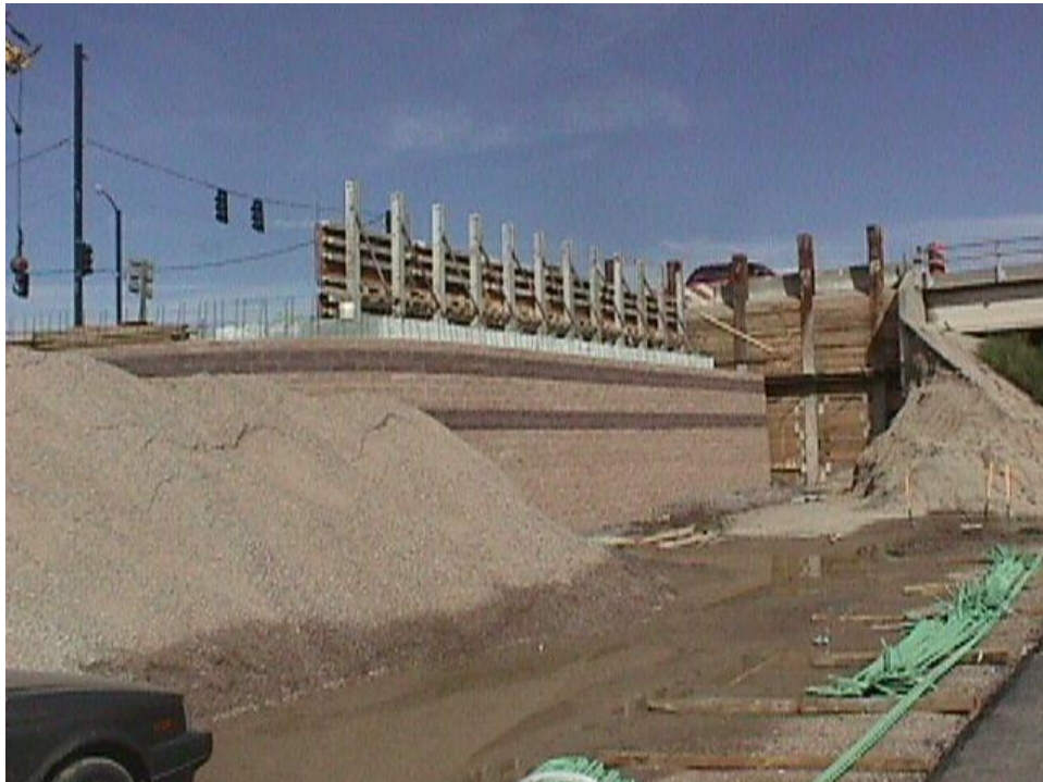
Figure B-26. The abutment wall footing has been poured and the forms are being set for the abutment wall.
