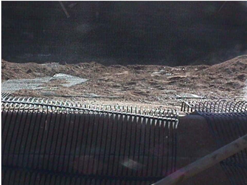
Figure B-16. Around the corners of the lower MSE walls, where geogrid from the front and side of the structure overlapped, a thin layer of fill material was placed between these geogrid layers to provide friction between them.
