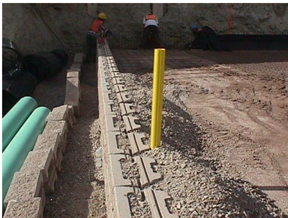
Figure B-4. Picture showing facing blocks, crushed stone used to fill in and 0.3 m behind the blocks, and the compacted CDOT Class 1 backfill. The yellow inclinometer tube was used to measure lateral movement in the structure along Section 400.
