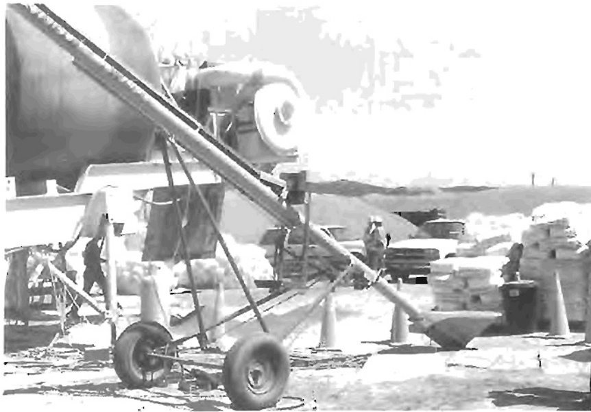
Figure 5. Auger system initially used for Vestoplast S
