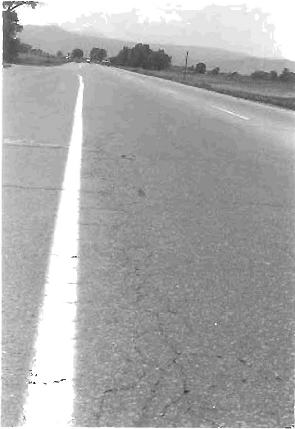
Figure 3. Overview of existing pavement.
