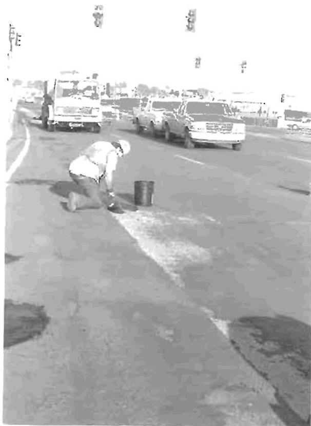
Figure 20. A cold-pour material was used to cover the area where the membrane was removed.
