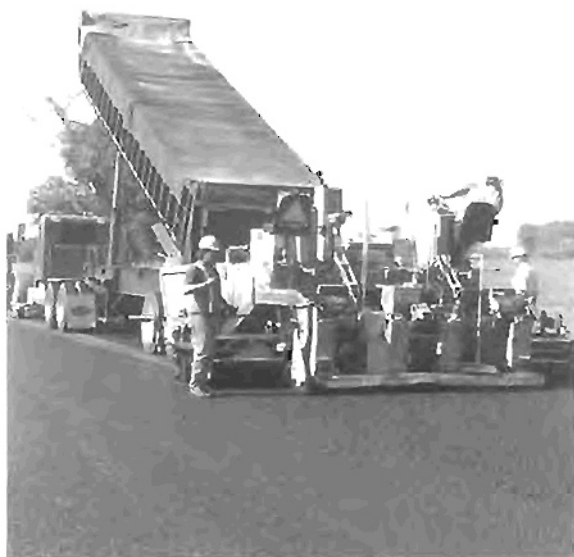
Figure 7. Typical laydown operation
