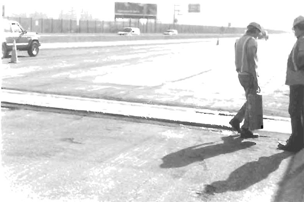
Figure 22. Preparing the joint prior to SMA placement.
