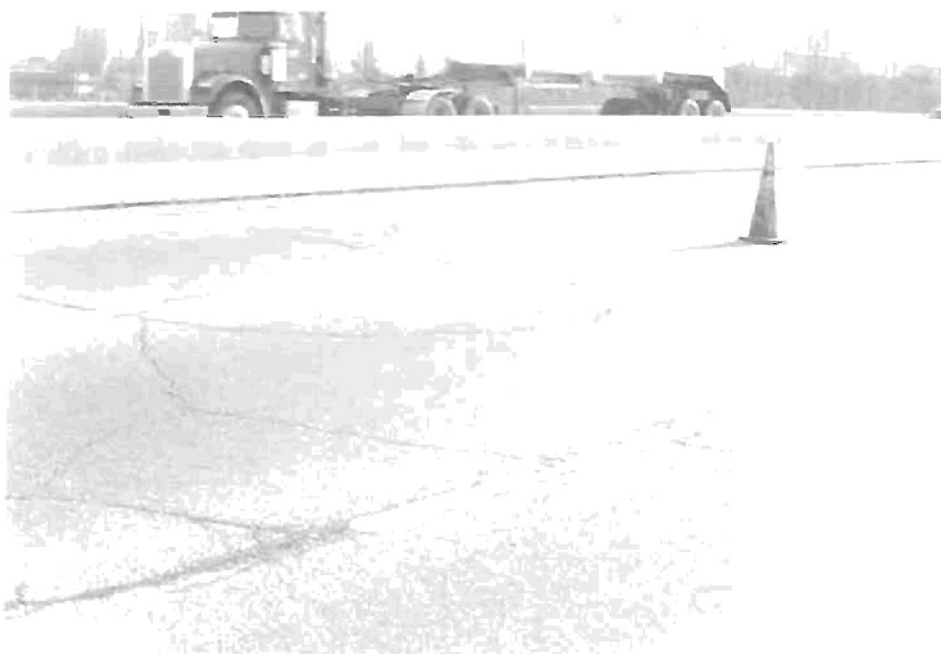
Figure 17. Typical cracking pattern prior to paving.
