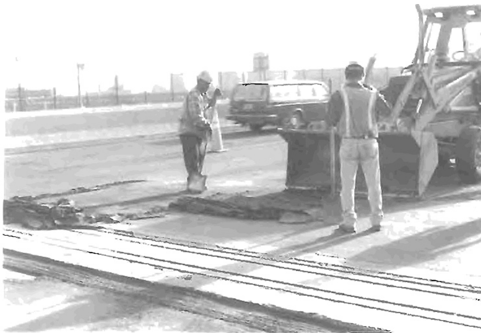
Figure 21. Removing the taper at the expansion joint.
