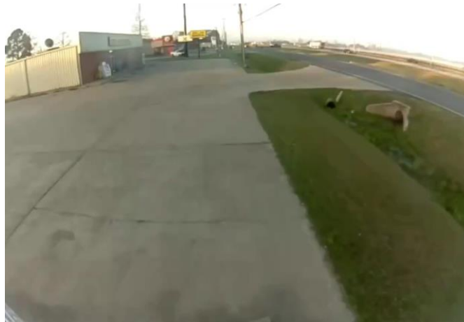
Figure 144. Camera view at LA 1 South entrance/exit
