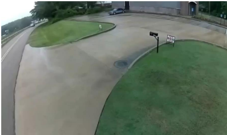
Figure 156. Camera view at Service Rd West entrance/exit
