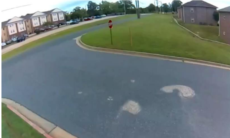
Figure 134. Camera view at Goyne St entrance/exit
