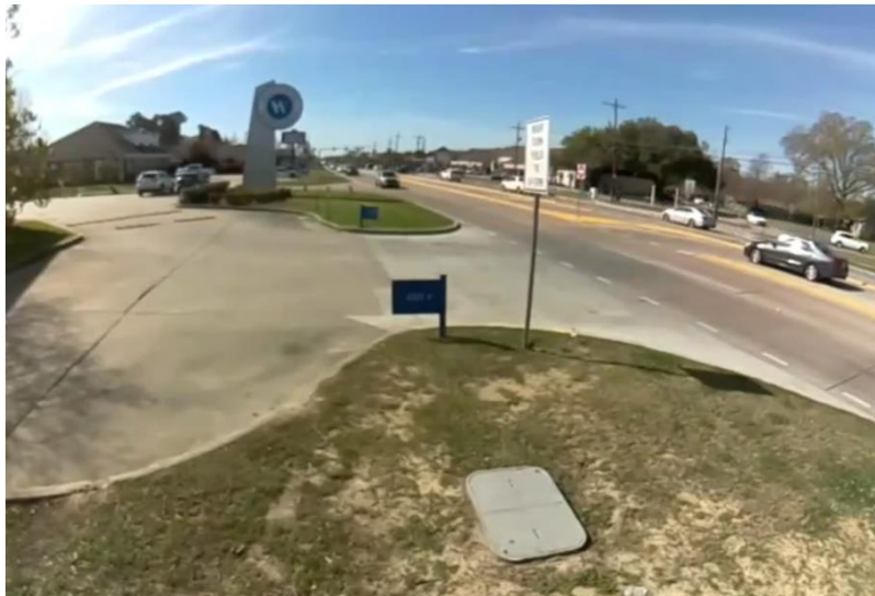
Figure 138. Camera view at South Range Ave entrance/exit (S1)
