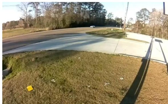
Figure 137. Camera view at U.S. Hwy 190 East entrance/exit
