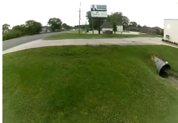
Figure 150. Camera view at Vincent Rd entrance/exit
