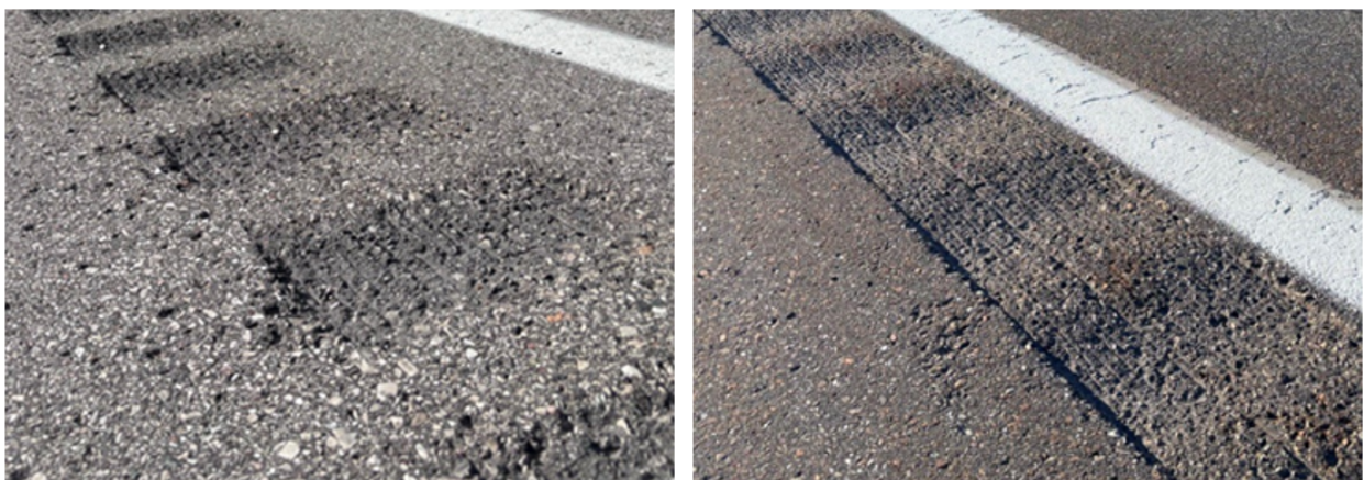
Figure 4. Traditional Rectangular (left) and Sinusoidal (right) Shoulder Corrugations
