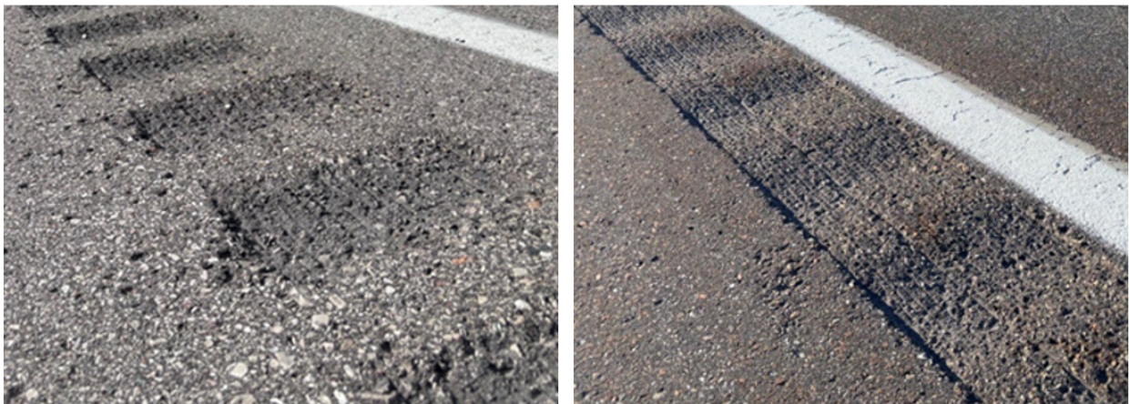
Traditional Rectangular (left) and Sinusoidal (right) Shoulder Corrugations
