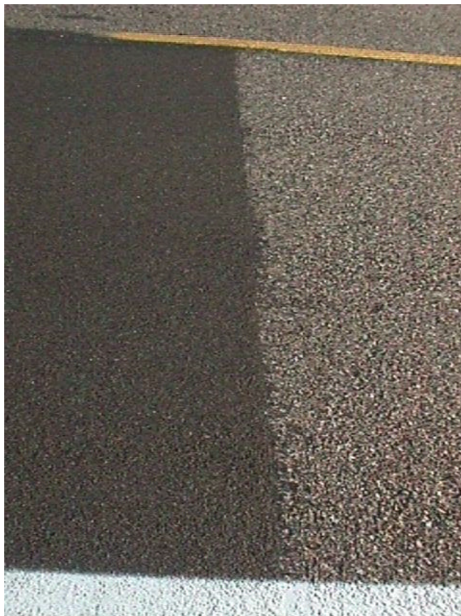
Figure 3. The light weight chip section at the east end of the site. The right lane is the light weight chip seal. The dark patch in the left wheel path is water left by the skid testing equipment.
