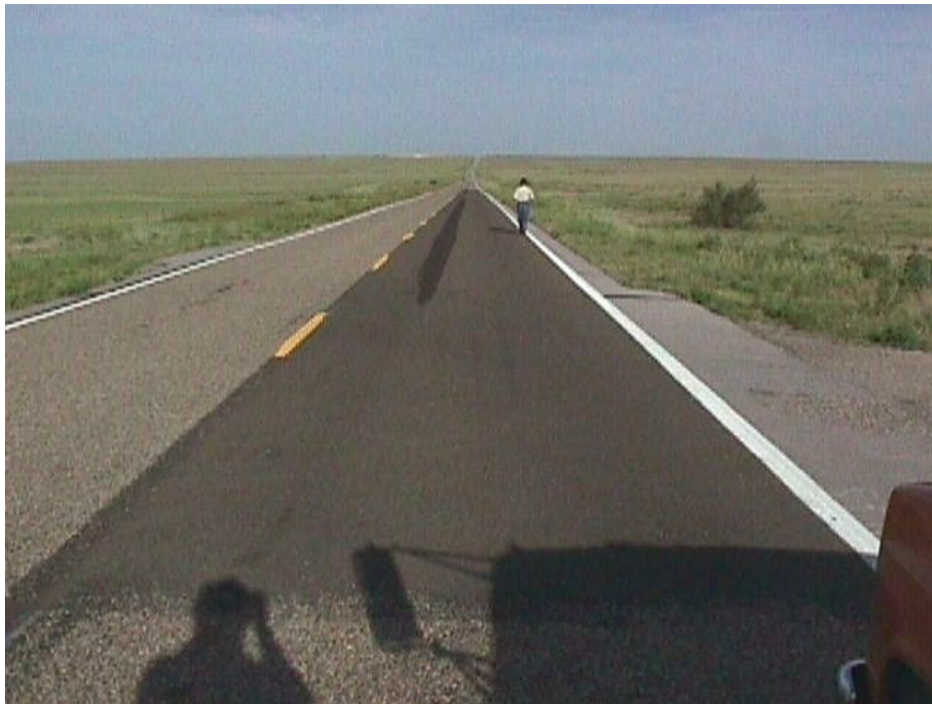
Figure 3. The light weight chip section at the east end of the site. The right lane is the light weight chip seal. The dark patch in the left wheel path is water left by the skid testing equipment.
