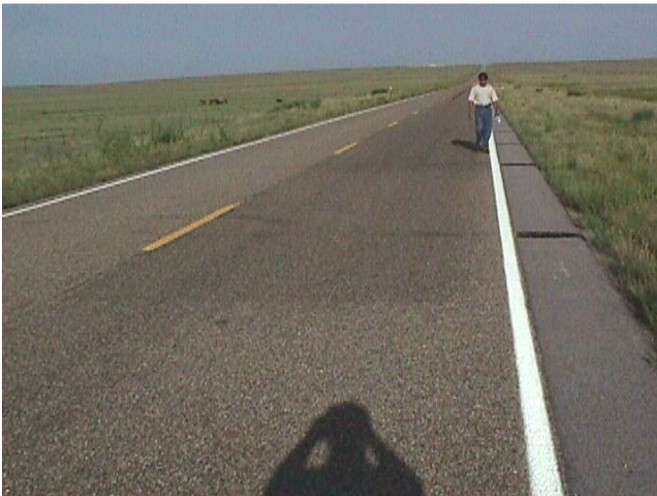
Figure 2. The fog seal section starts where the pavement is darker. The dark stripes on the shoulder are seals applied to transverse cracks before the chip seals were placed.
