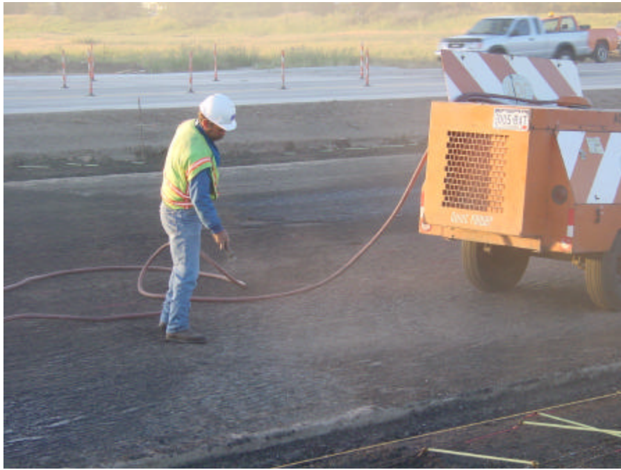
Figure 31. Air Blasting Asphalt Surface Prior to Concrete Placement
