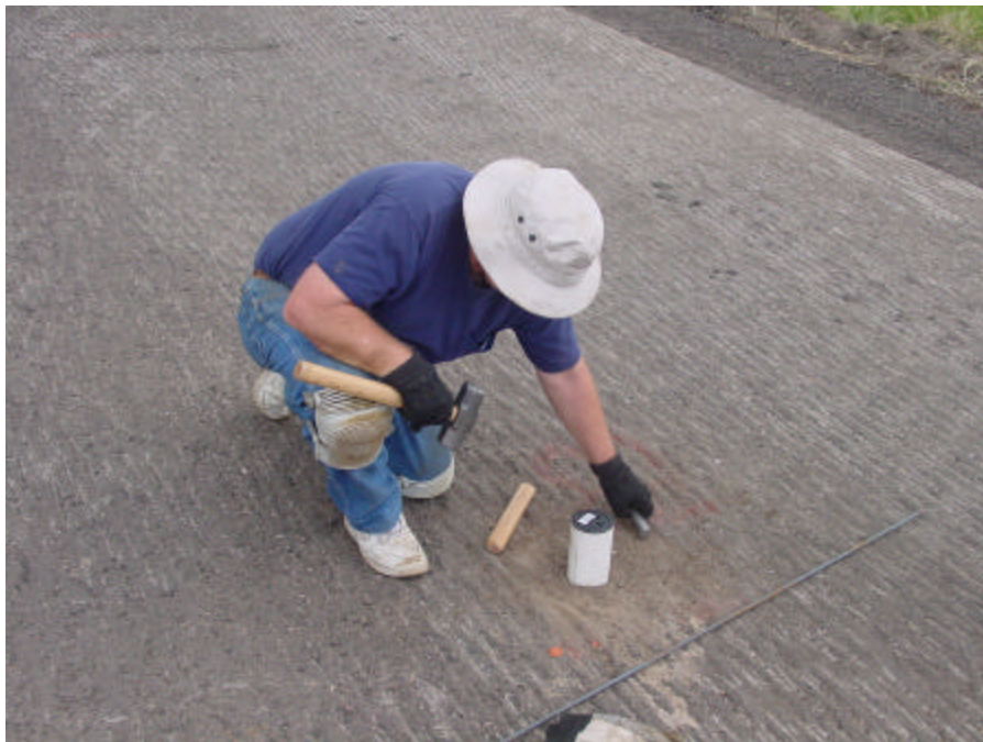
Figure 18. Completed Reference Rod Installation
