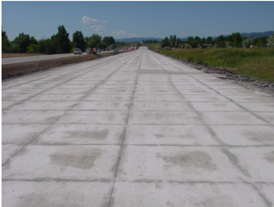
Figure 38. Pavement Surface After Joint Sawing
