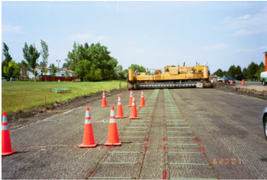
Figure 33. Tie Bar Assembly for Test Section 1
