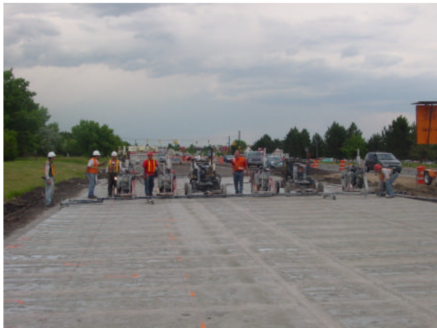
Figure 36. Sawing Transverse Control Joints
