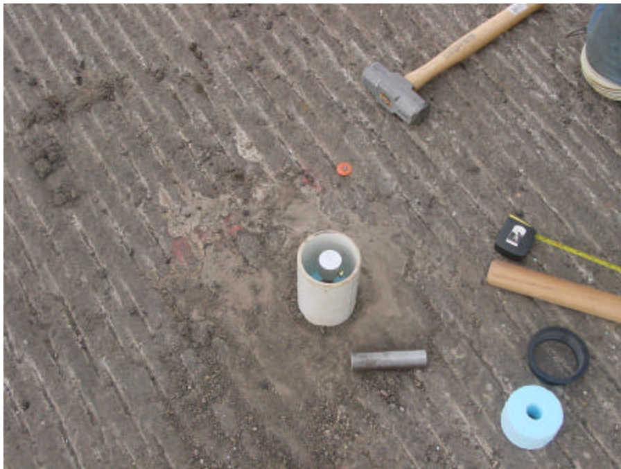
Figure 17. Installation of Reference Rods, continued
