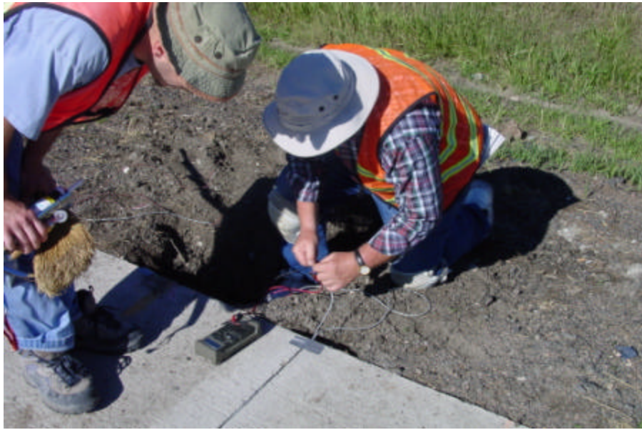
Figure 27. Checking Installed Gages
