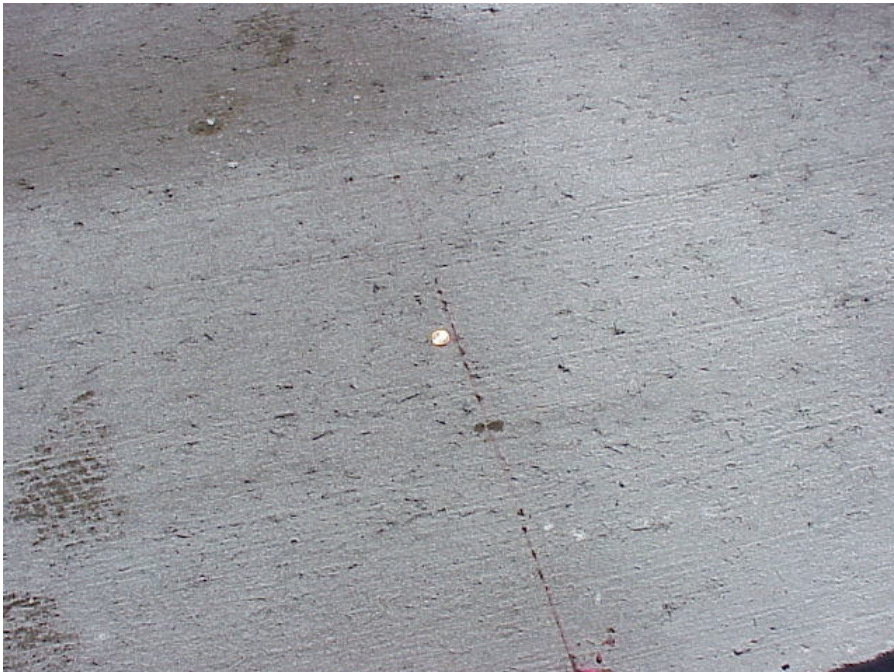
Figure 35. Surface Texture Provided by Astroturf Drag
