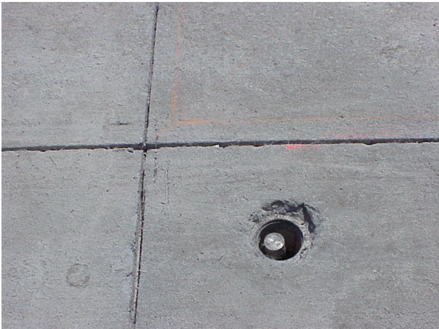
Figure 38. Pavement Surface After Joint Sawing
