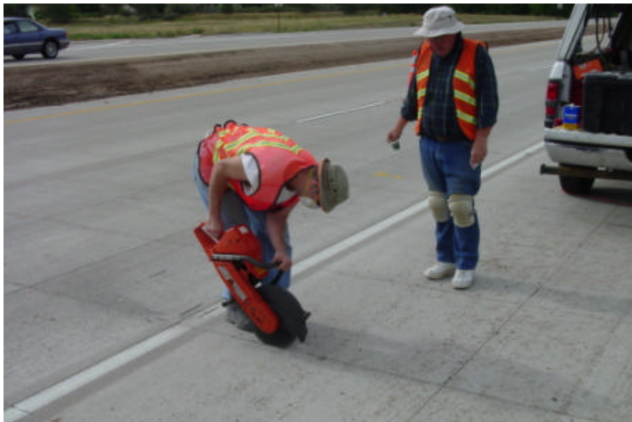
Figure 24. Cutting Grooves Along Joints for Gage Cables
