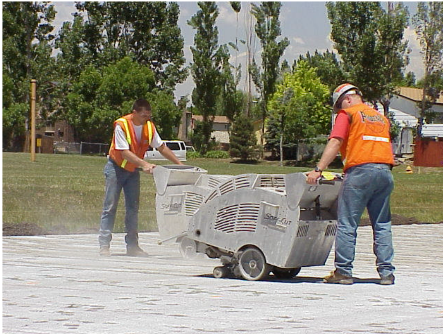
Figure 36. Sawing Transverse Control Joints
