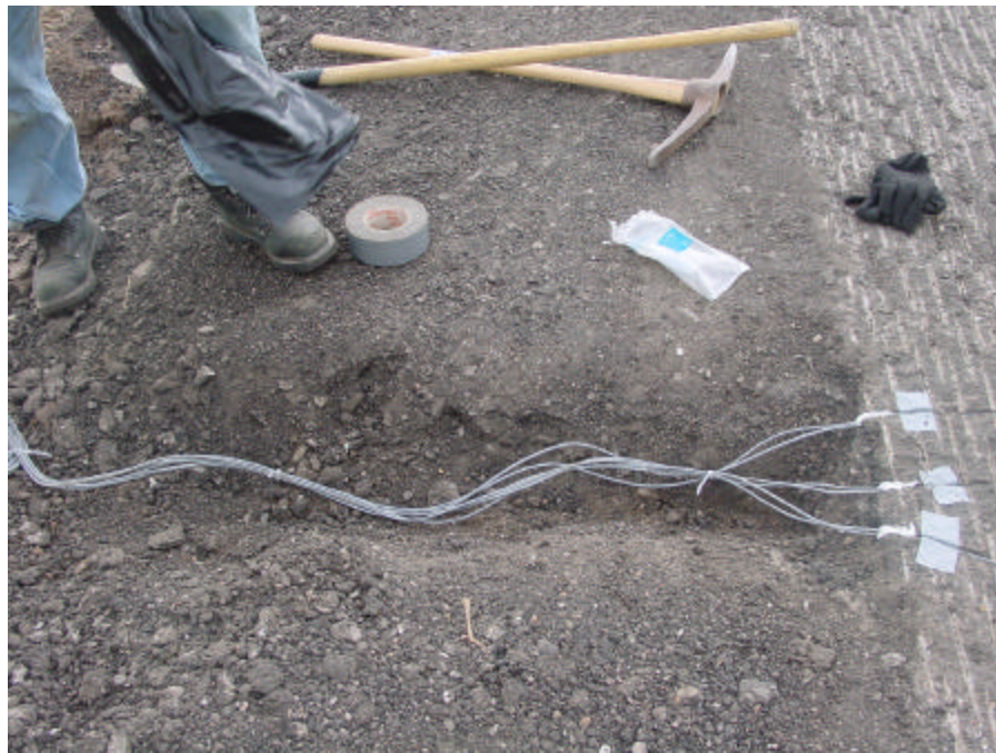
Figure 15. Recess and Protection of Lead Wires
