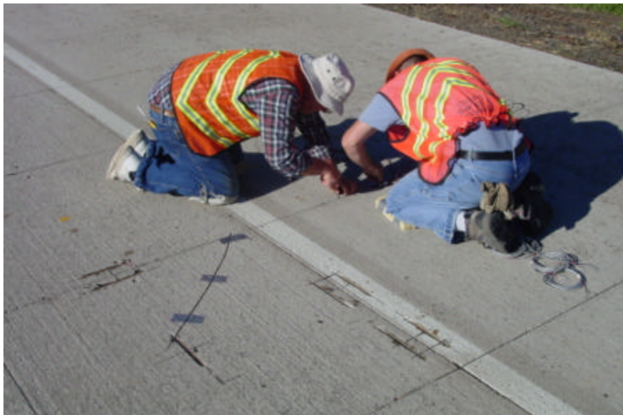
Figure 26. Recessing Leads
