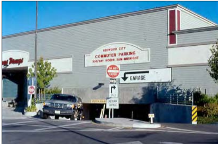
Figure 3j. Parking Facility at Station Area
