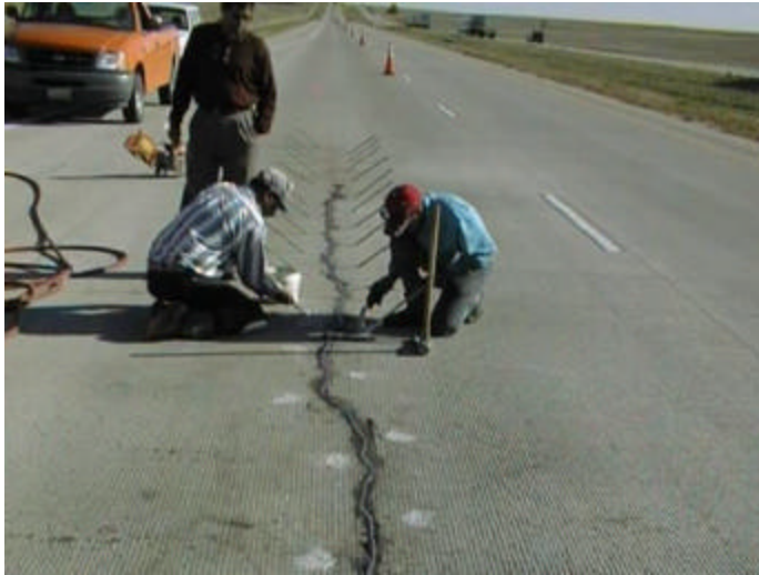
Figure 4. Installation of stitches on I-70 at Agate.
