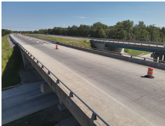
(a) Upper-side view of the bridge
