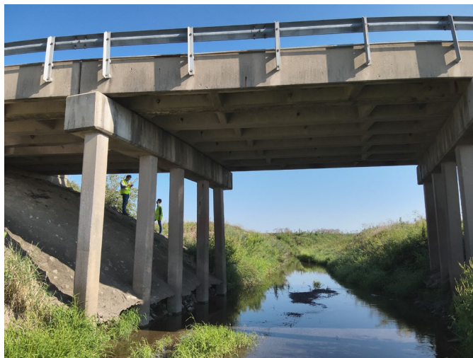
(b) Bottom-side view of the bridge
