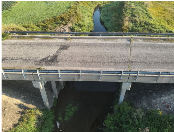
(a) Upper-side view of the bridge
