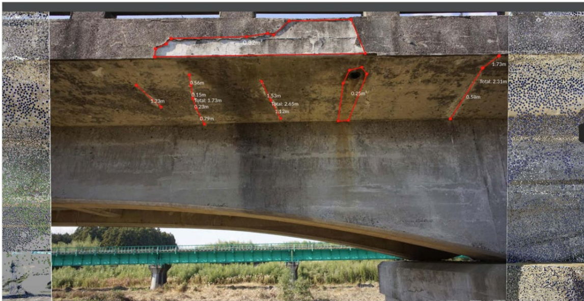
Figure 22. Illustration. Demonstration of defect measurement in a virtual inspection environment.
