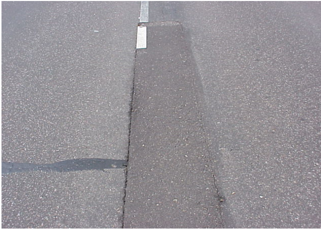
Figure 24 – This photo shows the initial longitudinal joint crack on the left. Then the contractor milled and filled one foot to the right of the crack. Eventually this pavement cracked on the edge of the 1-foot mill and fill, creating 2 cracks.
