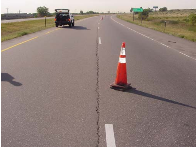
Figure 14 – Longitudinal construction joint failure at end of warranty period. Longitudinal crack is evident throughout most of the project.
