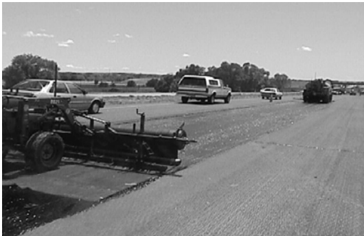
Figure 6 – Placement of Petromat material.
