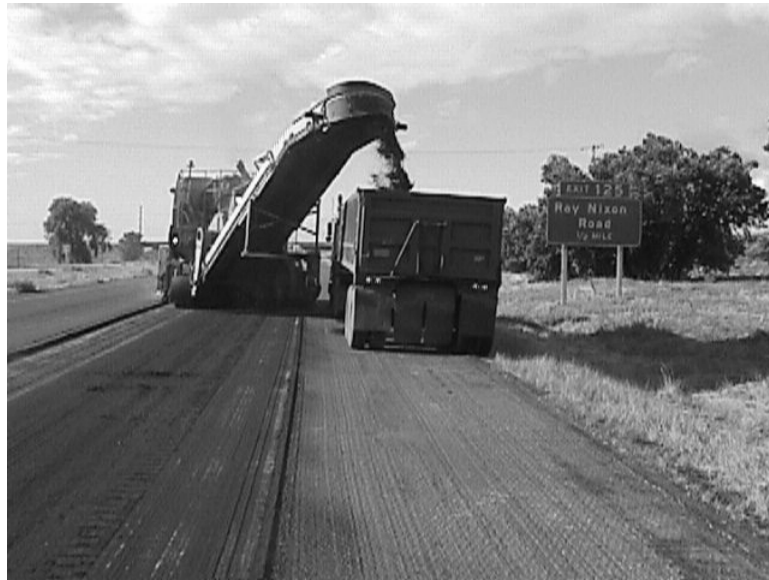
Figure 2 - Rotomilling operation.
