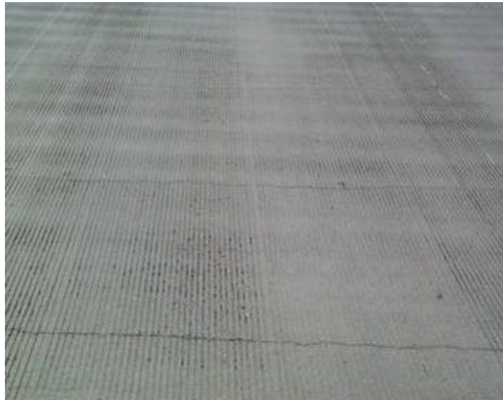
Figure F.3 Crack pattern at the mid-span (3.5 ft spacing)
