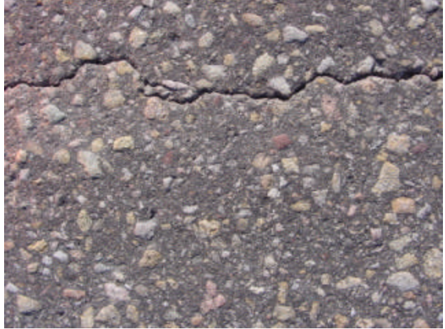
Top-Down Cracking
