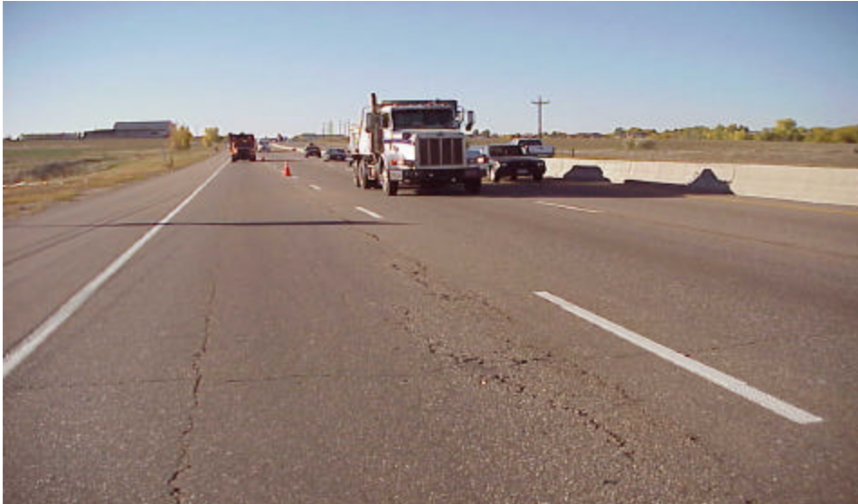
Figure 1. Longitudinal cracking was found on this project as shown in this photograph. This cracking pattern was consistent throughout the entire length of the project.
