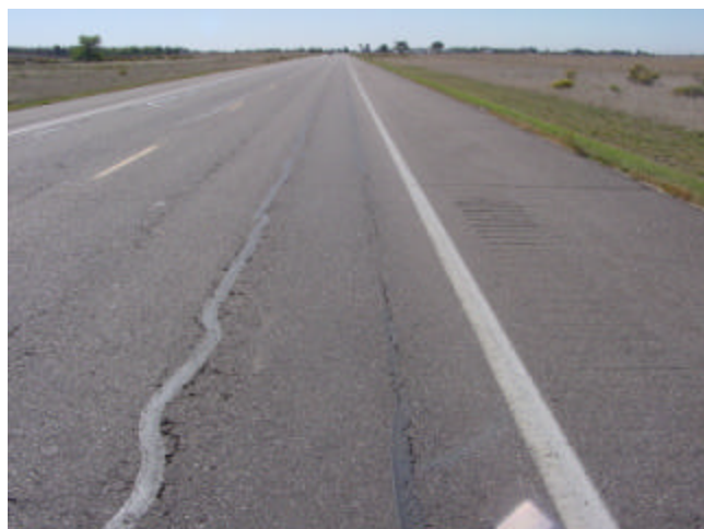
Top-Down Cracking
