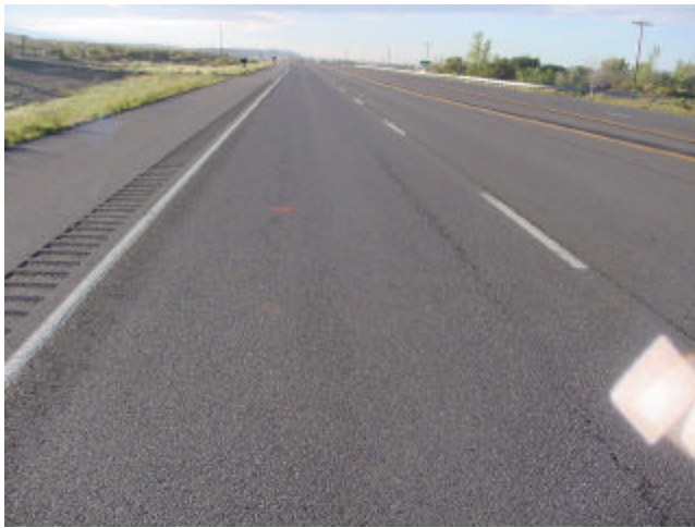
Top-Down Cracking
