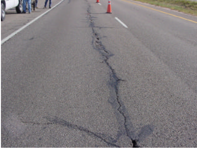
Reflective Cracking
