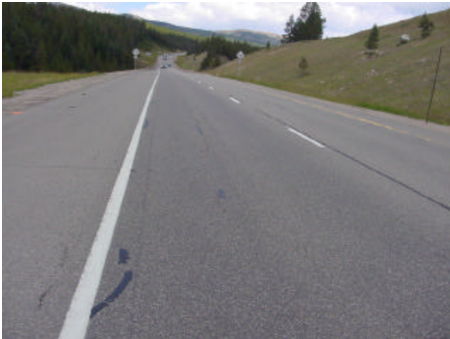
Top-Down Cracking
