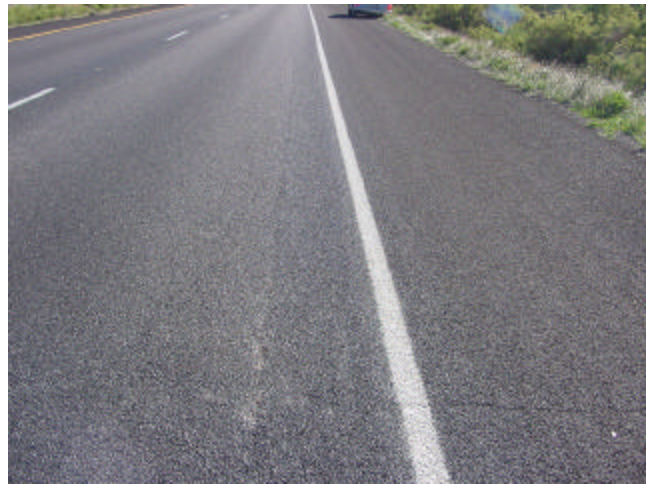
Top-Down Cracking
