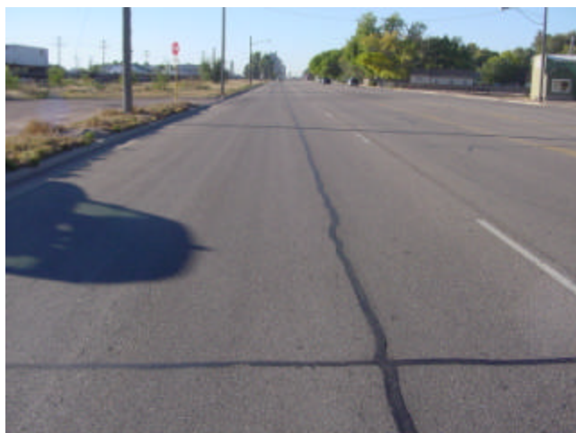
Top-Down Cracking
