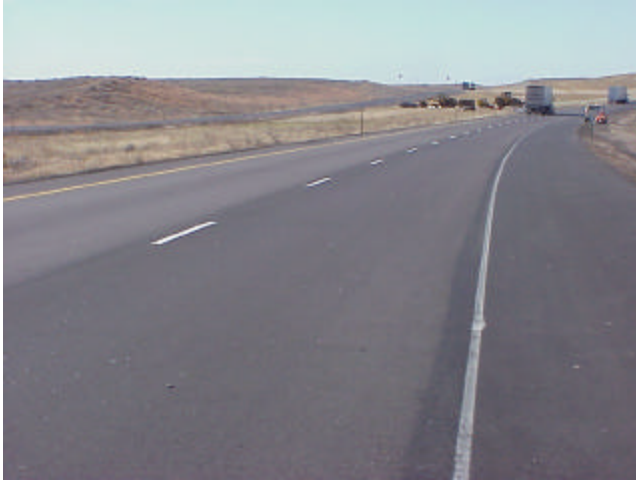
Figure 10. This photograph shows the project shortly after construction. Segregation on the surface was not apparent.
