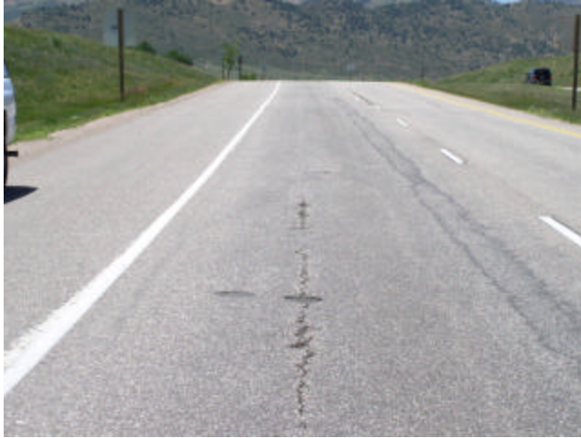
Top-Down Cracking
