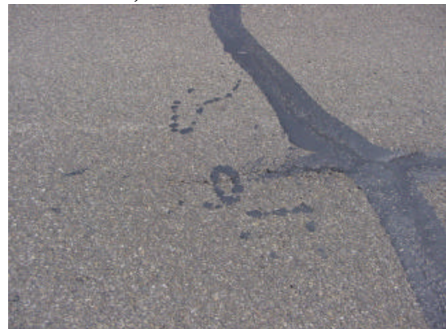
Reflective Cracking
