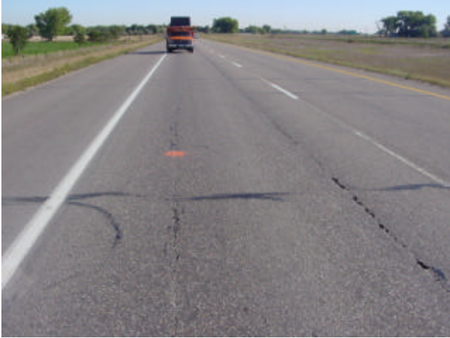
Top-Down Cracking
