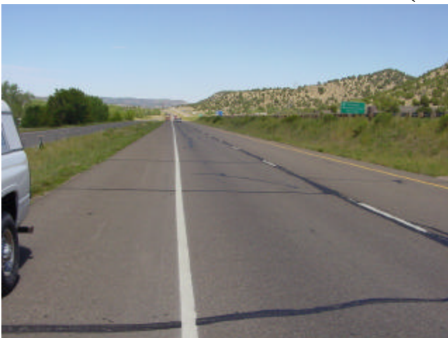
Reflective Cracking
