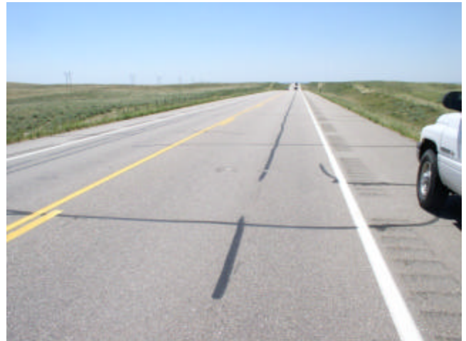
Reflective Cracking
