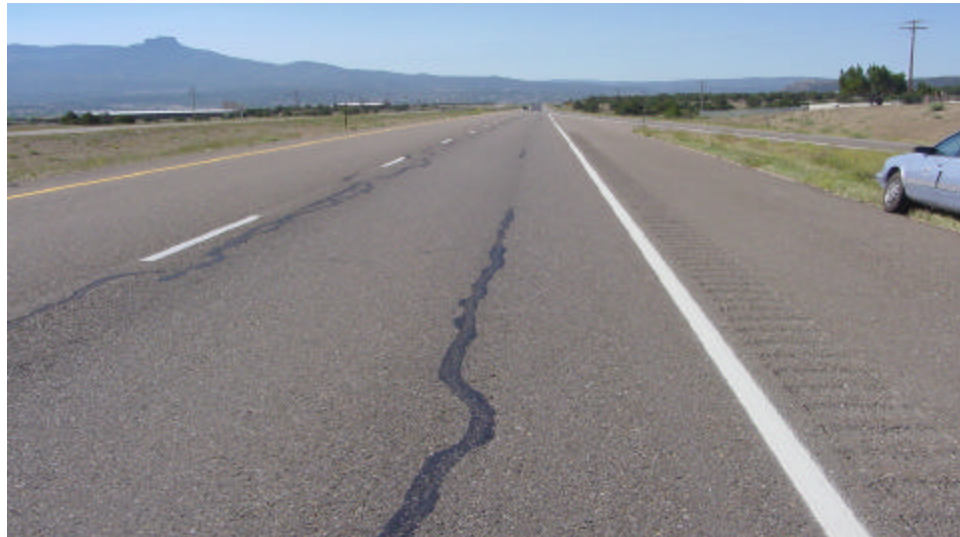
Figure 15. This crack was top-down. Although the crack is straight, the severity was enough to warrant crack sealing.
