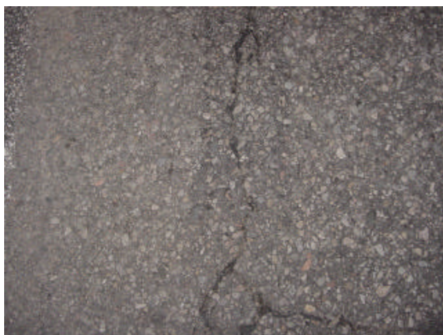
Reflective Cracking
