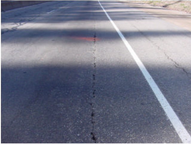
Top-Down Cracking
