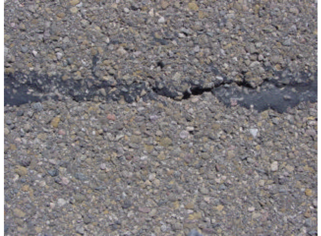
Top-Down Cracking
