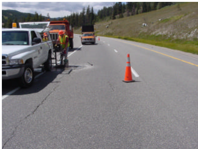
Top-Down Cracking
