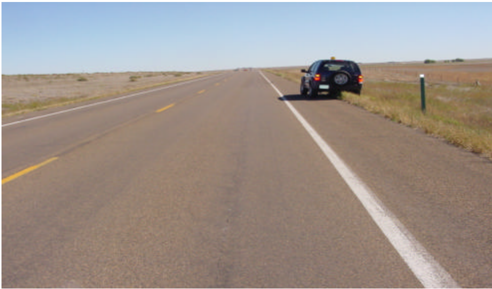
Figure 14. This distress was a reflective crack. Note the linear straightness and low severity of the crack.
