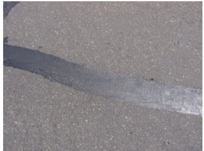
Reflective Cracking
