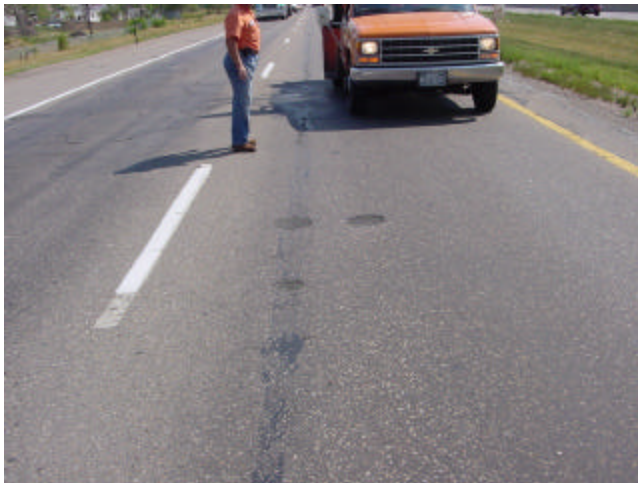
Top-Down Cracking
