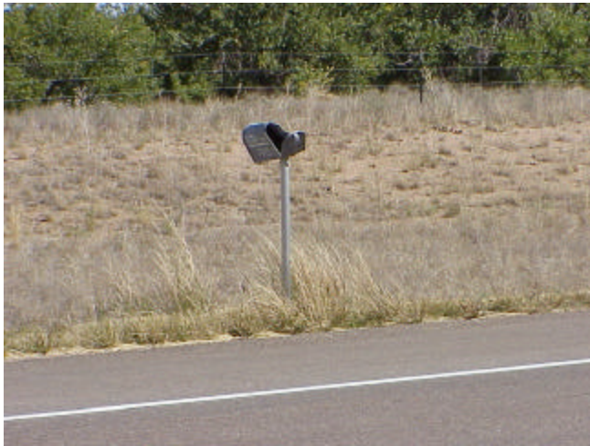
Figure 1. Mailboxes mounted near high-speed highways are susceptible to damage from the blast of snowplow during the winter.
