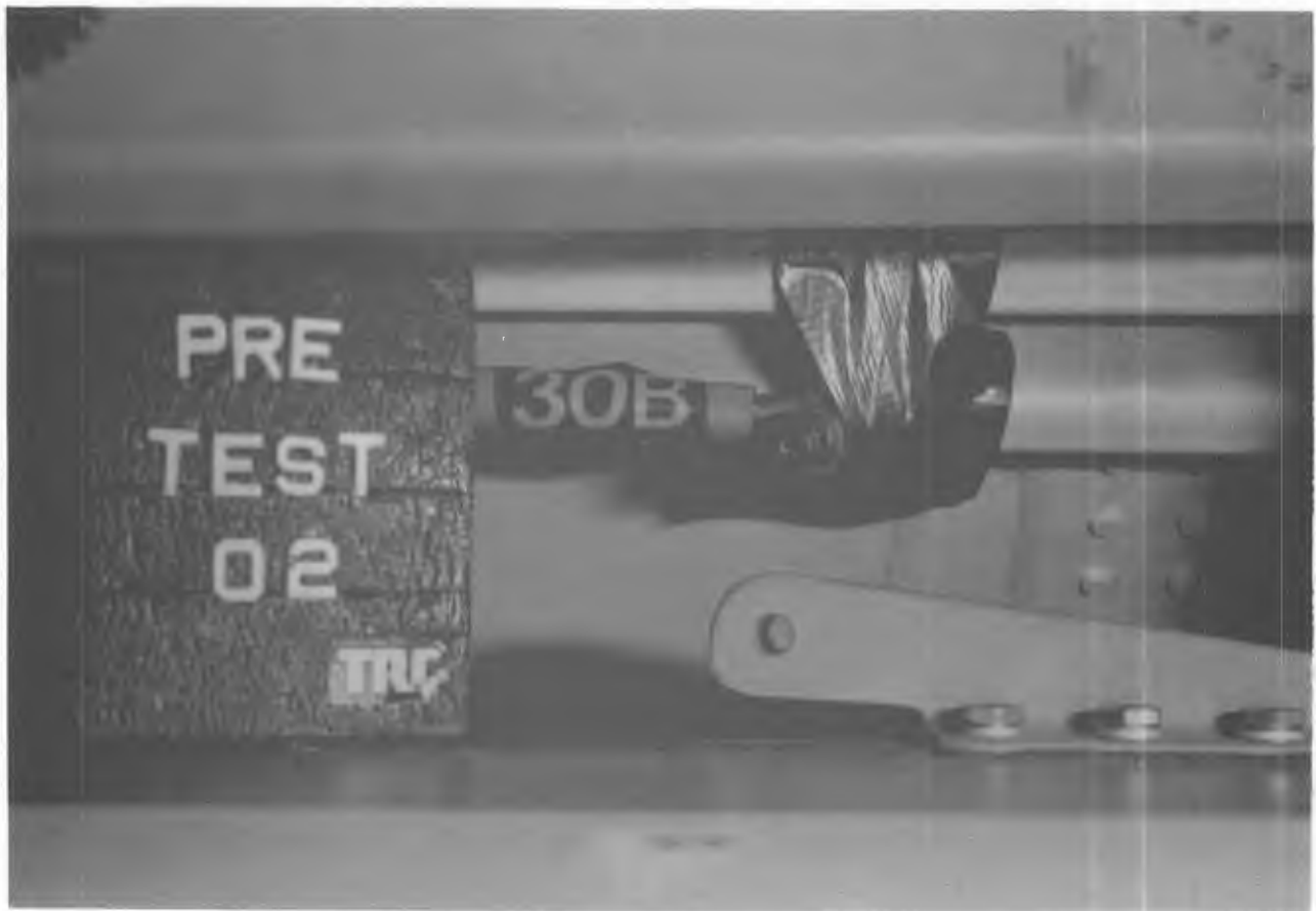
Figure C-17. PRE-TEST OHBC-02, BIN 'B' LINK 30 DETACHED C-19
