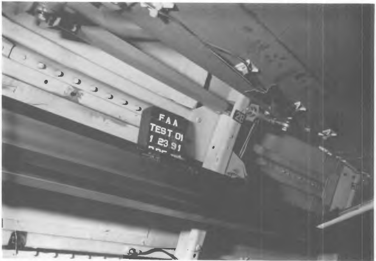
Figure 18. PRE-TEST BIN 'B' LINK 2
