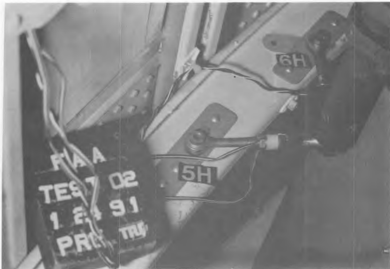
Figure 93. PRE-TEST BIN 'A' LINKS 5 AND 6
