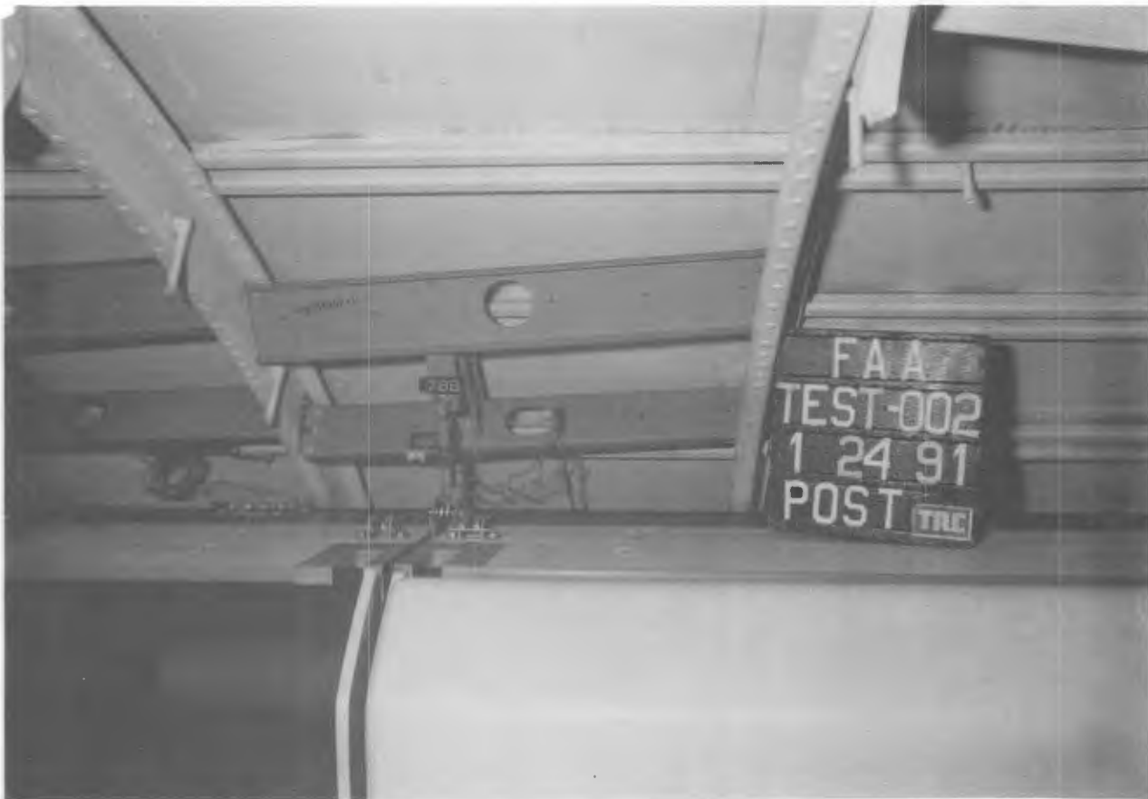
Figure 101. POST-TEST BIN 'B' LINKS 18 AND 25
