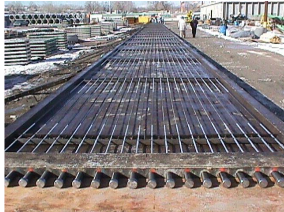
Fig. 3.6 Prestressing bridge decks using CFRP
