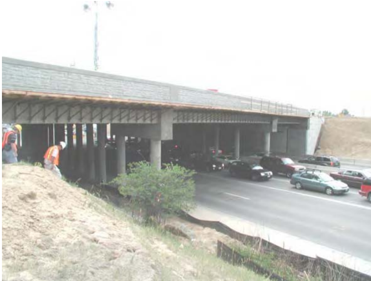
Fig. B1.2.1 Bridge on I-25 over Orchard
