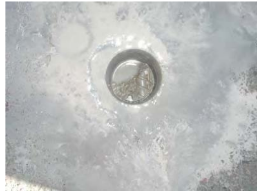
Fig. C.3.9 An epoxy-coated rebar in good condition
