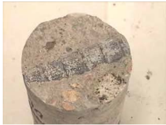
Fig. C.1.13 An extracted steel rebar – in good condition
