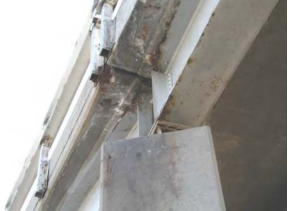
Fig C.1.5 Efflorescence and corrosion damage on the lower elevation (slope) of the bridge
