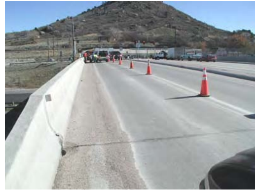
Fig. C.3.3 The bridge surface of Wolfensburger over I 25
