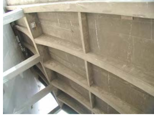
Fig. C.8.3 The bottom view of the girder system
