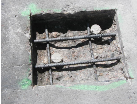
Fig. 3.3 The Galvashield cathodic protection system installed in SH 85 SB in Greeley, Colorado.
