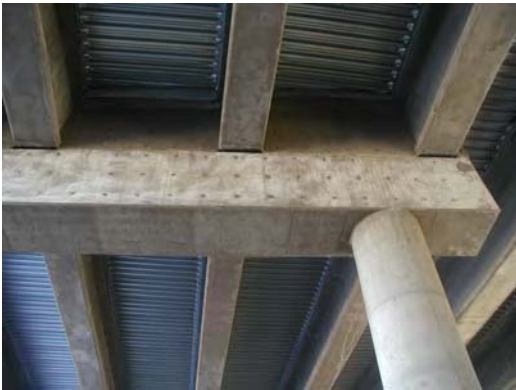
Fig. C.4.4 A bottom view of a pier cap and girder systems
