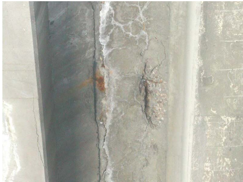
Fig. B1.5.2 Cracking and efflorescence on the bottom deck
