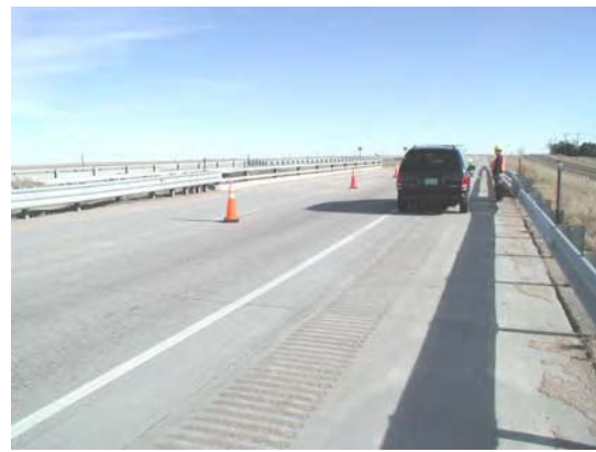
Fig. C.6.3 The surface of F-18-AQ structure
