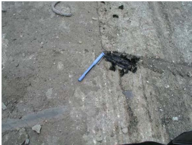
Fig. B1.2.2 Asphalt with membrane overlay
