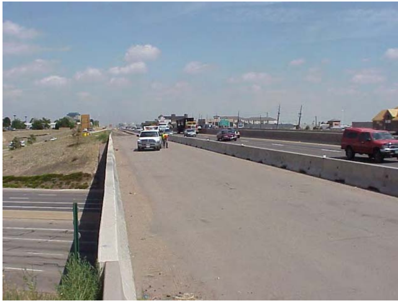
Photo A.3.3 Bridge deck – asphalt overlay
