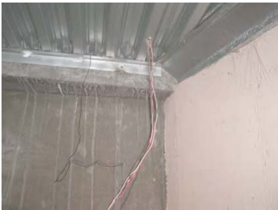
Fig. C.5.4 The wires of the corrosion monitoring system
