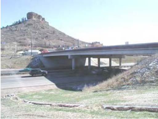
Fig. C.3.2 Wolfensburger bridge over I25
