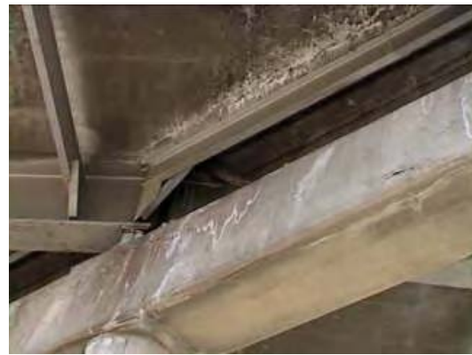
Fig C.1.9 Salt deposited on the pier cap and connection between girder and deck
