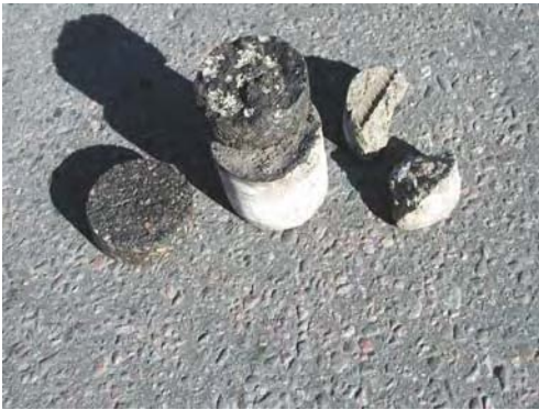
Fig. C.9.6 Concrete cores extracted from the driving lane
