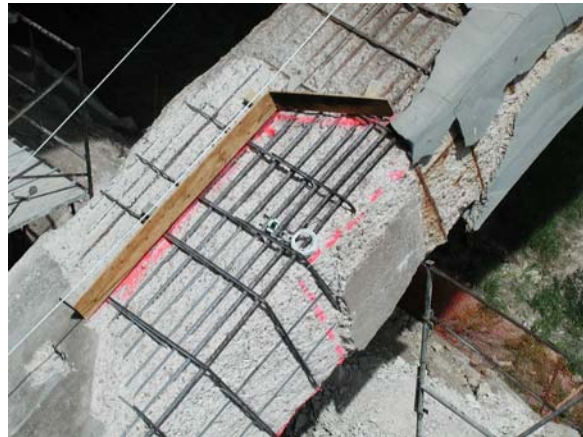
Fig. 3.2 Repair corrosion damage on the arch
