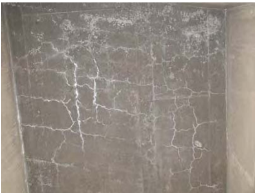
Fig. C.8.6 Efflorescence with crack pattern on the bottom of the slab (I)
