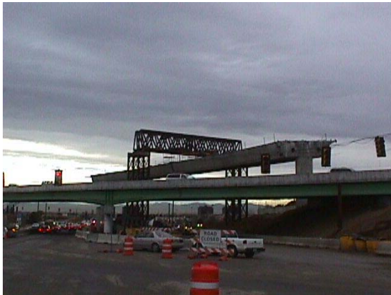
Fig. 3.5 I-225 & Parker Interchange project
