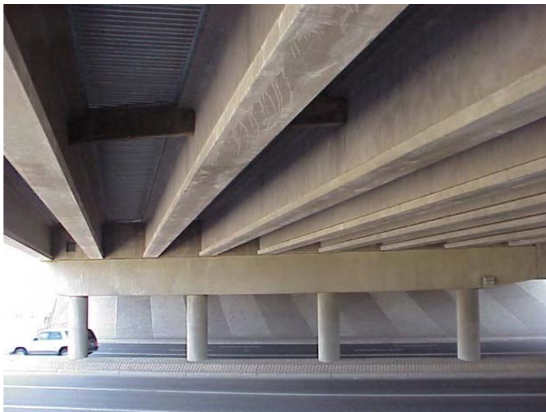
Fig. B1.3.2 Girder system – precast prestressed concrete
