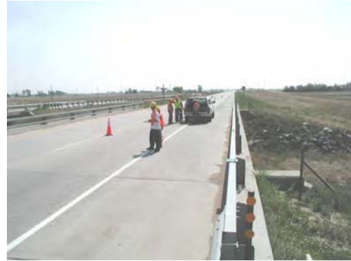
Fig. C.7.3 The bridge surface
