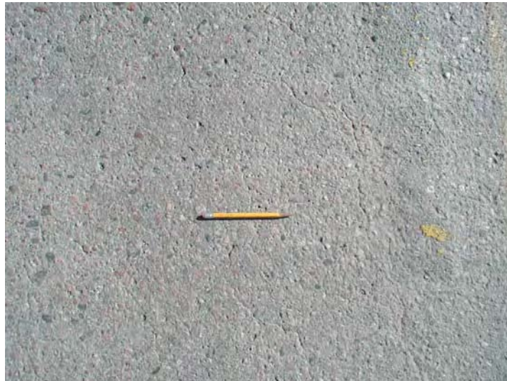
Fig. C.4.8 Transverse cracks
