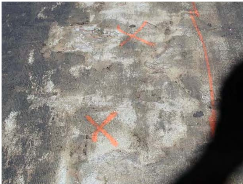
Fig. B1.4.2 A marked area of delamination on the deck – tested using hammer sound
