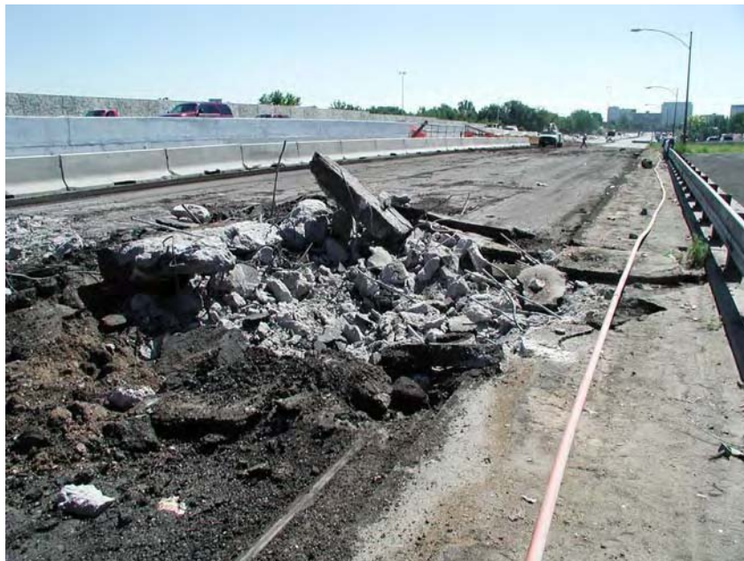
Fig. B1.7.6 Bridge decks under demolition process
