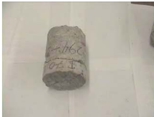
Fig. C.7.10 The delamination in the concrete overlay
