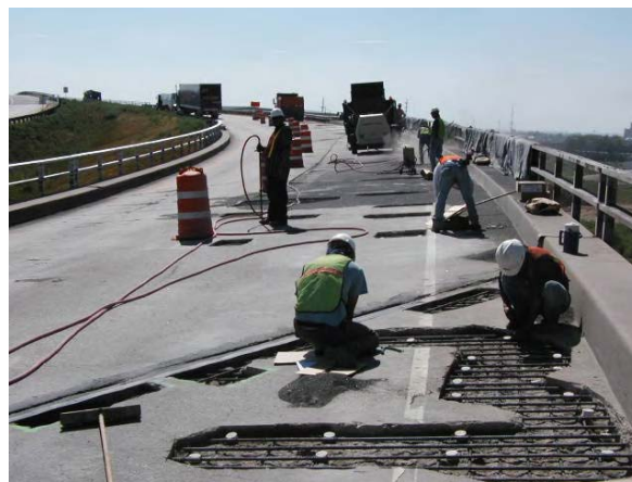
Fig. C.1.15. The Galvashield corrosion protection system installed on some parts of the bridge deck
