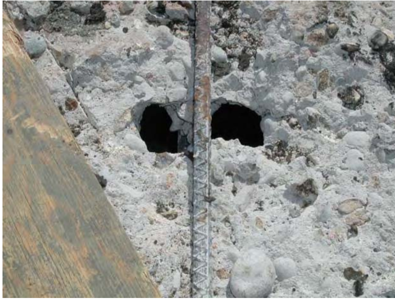
Fig. B1.4.3 Slab floor is heavily damaged (a big hole in the deck)
