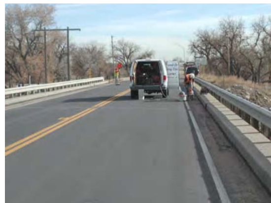
Fig. C.2.3 The bridge surface on SH 34 (New asphalt overlay with galvashield corrosion protection)
