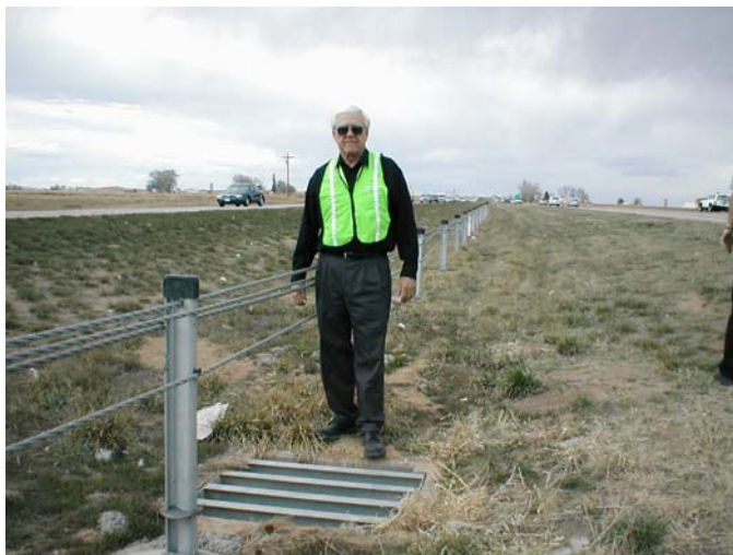
Figure 4. The cables over this drain inlet are much farther off the ground than the design specification.
