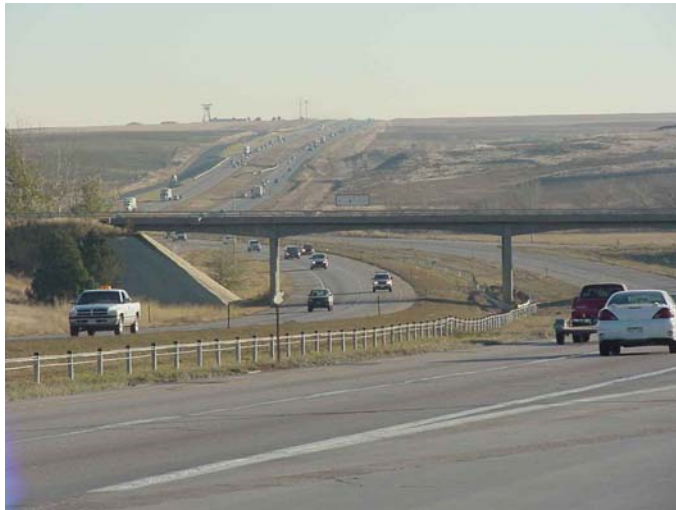
Figure 3. The I-25 – SH-56 interchange, looking south.
