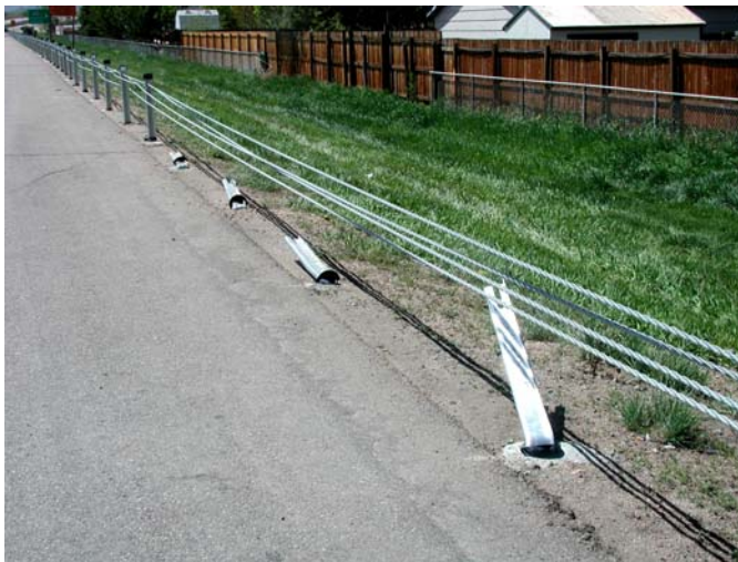
Figure 2. Only four posts were bent in this drive-away accident on US-285 at Kipling.
