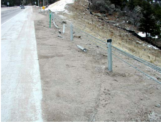
Figure 1. The most severe hit on the Windy Point systems damaged only six posts.
