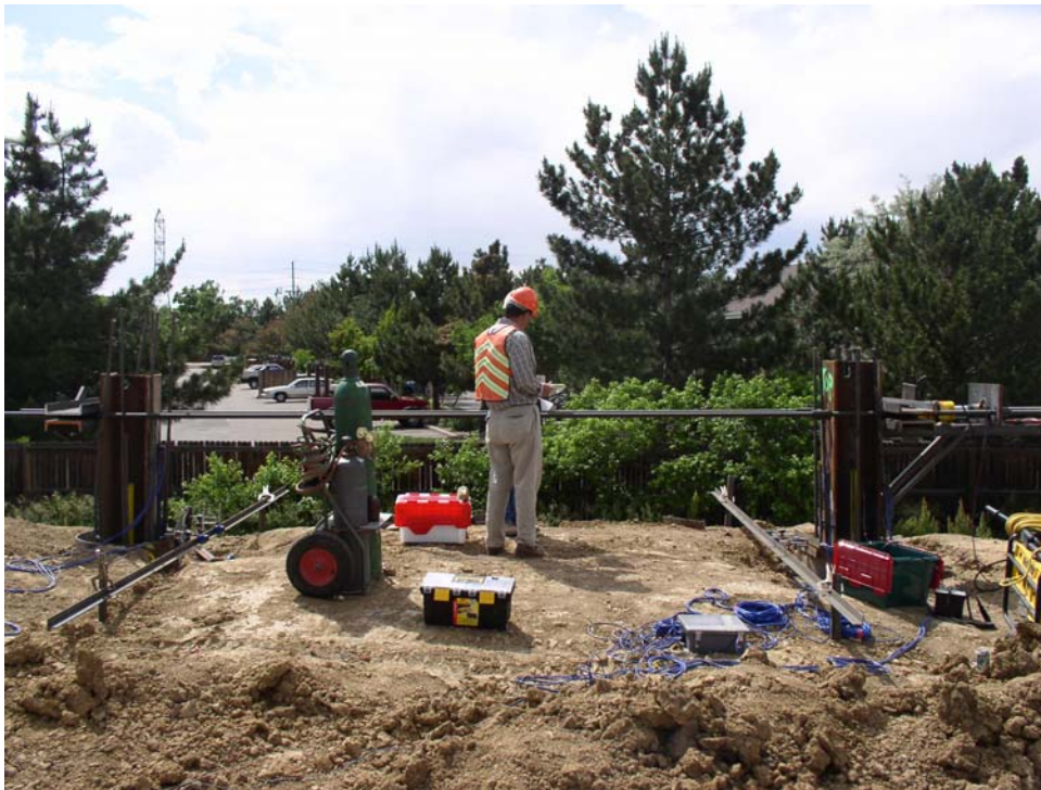
Figure 5.15 General view of the load test
