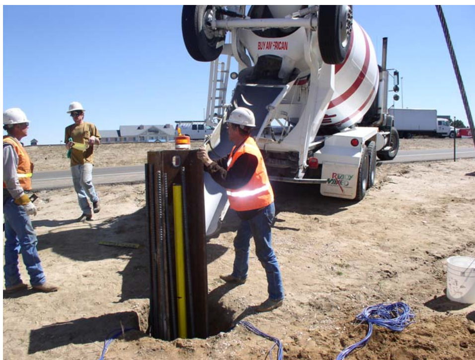
Figure 5.44 Drilled shafts installed and ready for concrete
