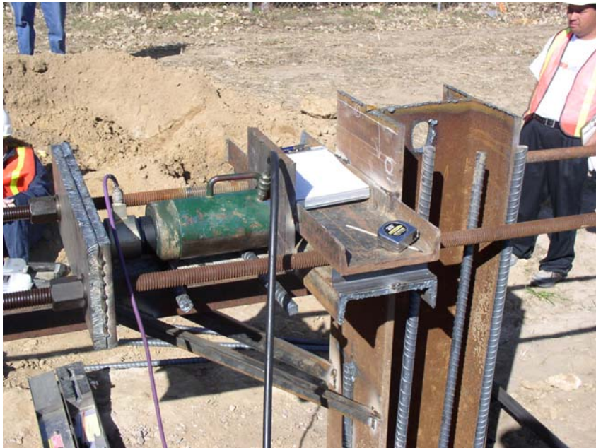
Figure 5.48 Picture showing the jacking devices
