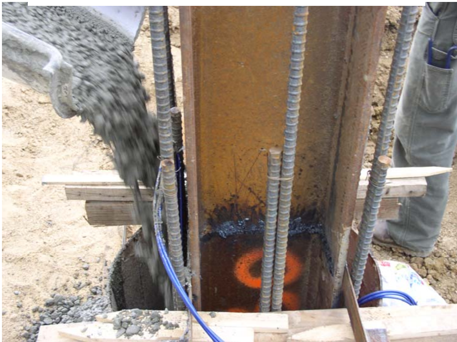
Figure 5.9 Pouring concrete in the hole
