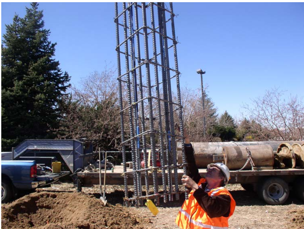
Figure 5.43 Instrumented cage transferred to the hole
