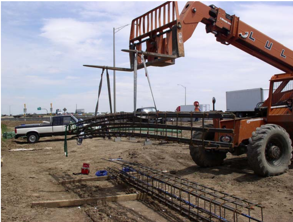
Figure 5.7 Instrumented cage transferred to the hole
