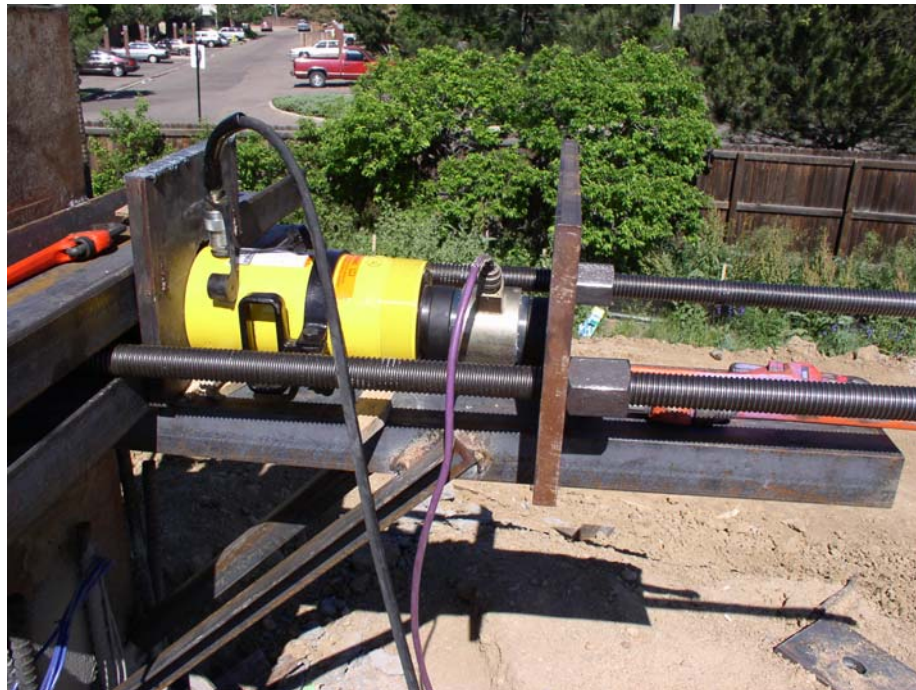
Figure 5.12 Picture showing the jacking devices
