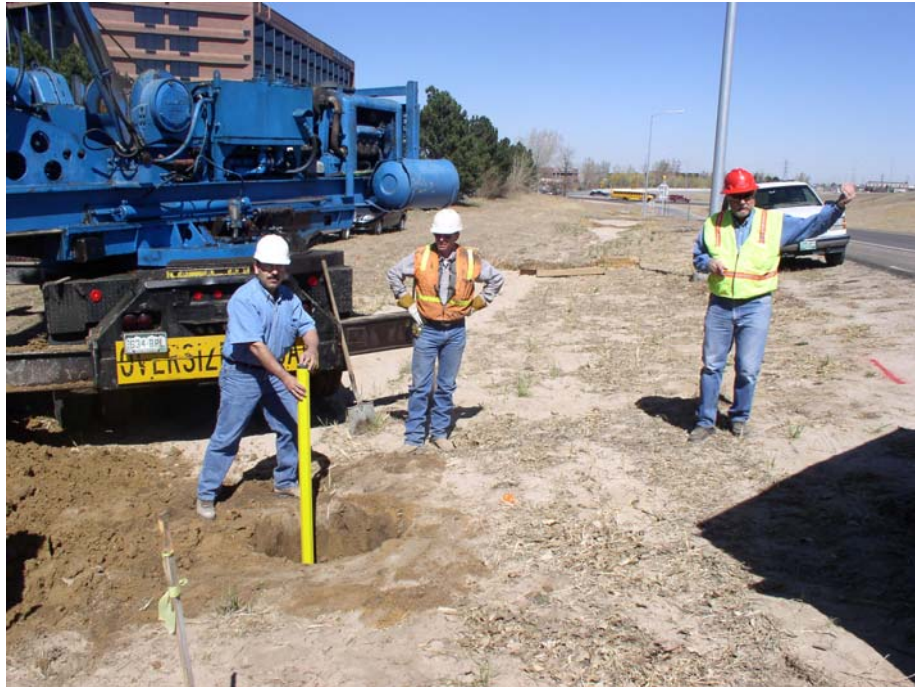
Figure 5.41b Inclinometer installation in the hole
