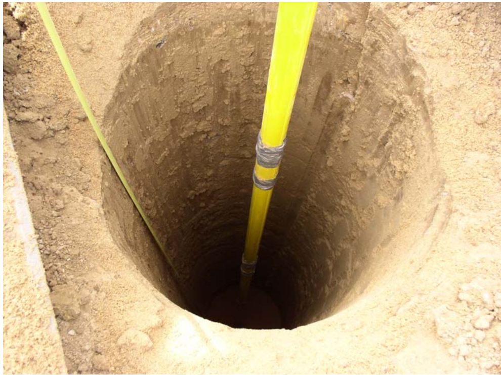
Figure 5.5b Inclinometer installation in the hole
