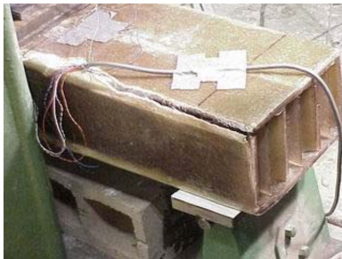
Figure 5-37 Failure mode in Test 3
