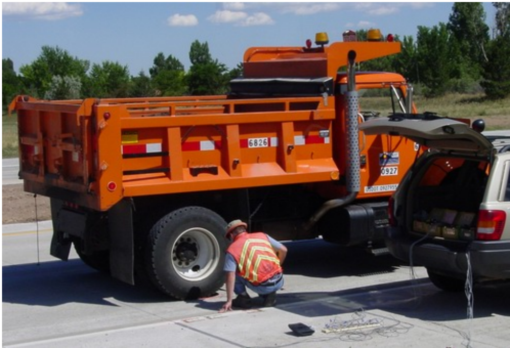
Figure 4.3. Truck Wheel Placement During Load Testing
