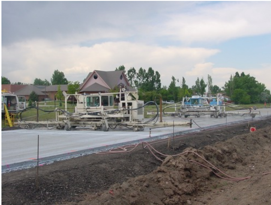
Figure C.3. Sawing Transverse Control Joints
