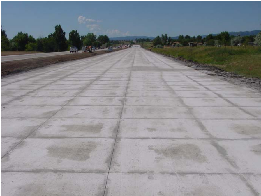
Figure C.5. Pavement Surface After Joint Sawing
