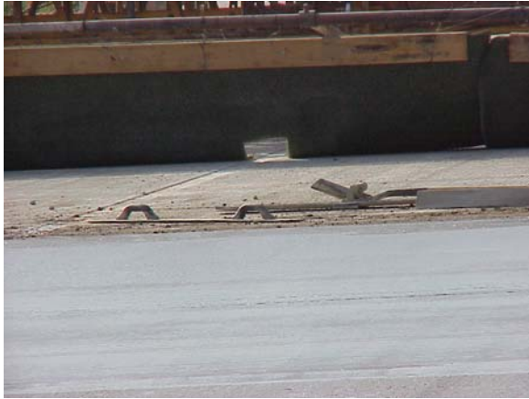
Figure 3. Gaps were cut in the drag to keep the groove smooth.
