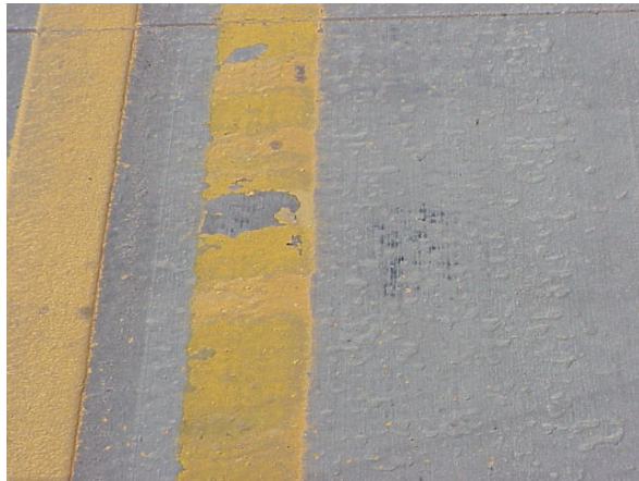
Figure 8. Epoxy paint in a groove in perfect condition next to damaged paint on the surface.
