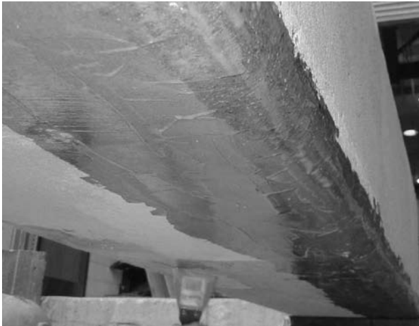
Step 1: Wetting surface with epoxy
