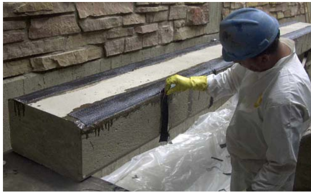
Figure 2-7 Placing CFRP sheet on concrete in progress
