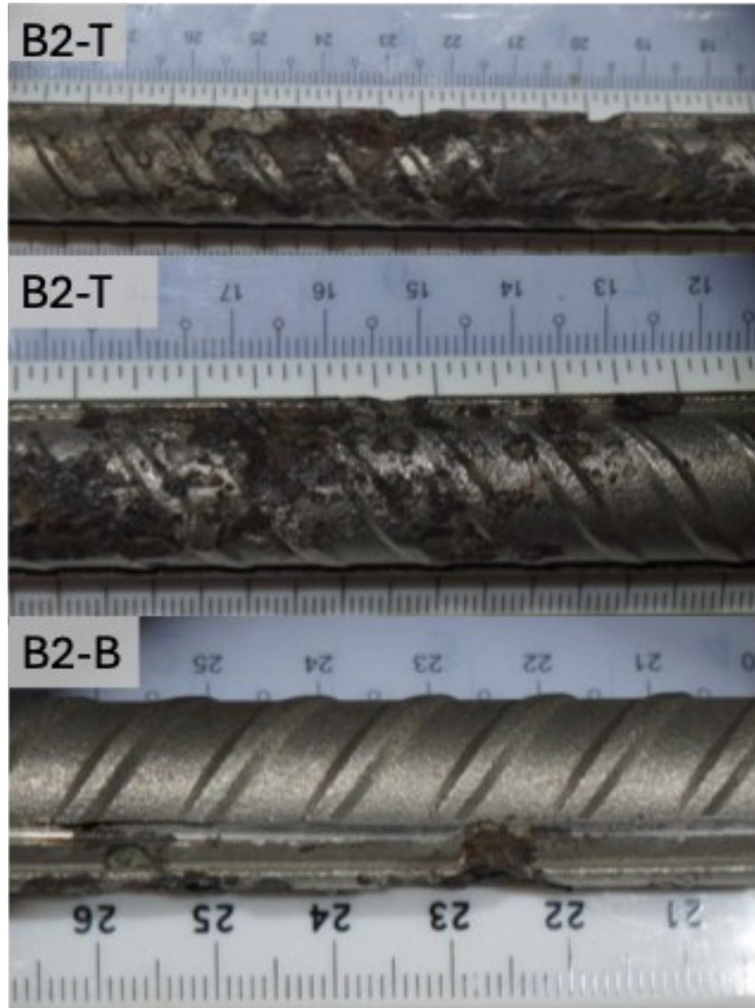
Figure 7-29. Rebar B2 closeups (top and bottom).
