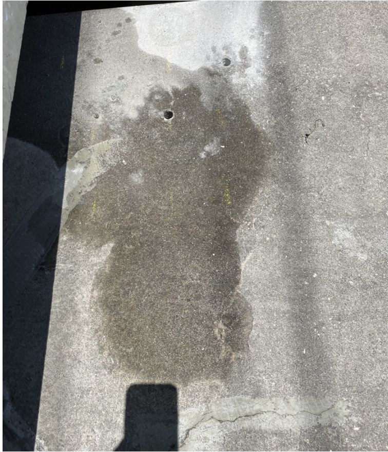
Figure 6-2. Drilled hole to access rebar at location one. A crack was visible transverse to the phone shade.
