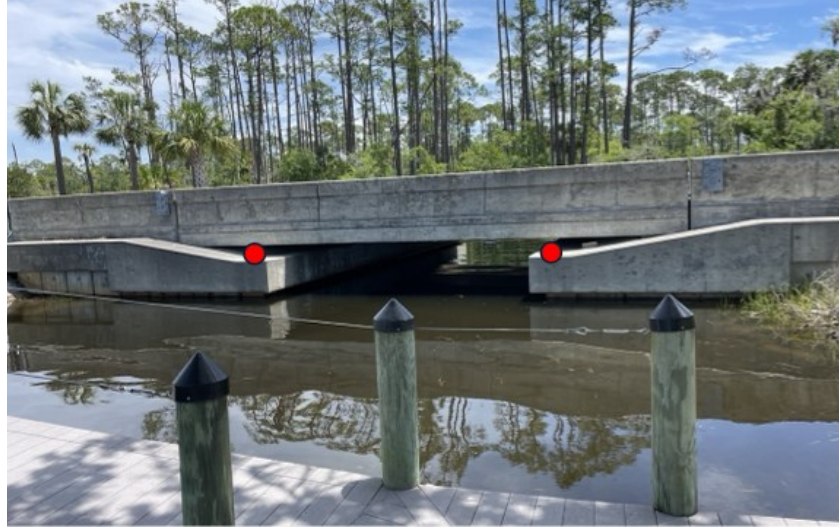
Figure 2-14. Picture of SR30A Bridge (#510072) taken from the marina. Left circle marker indicates drilling location 1; right circle marker indicates drilling location 2.
