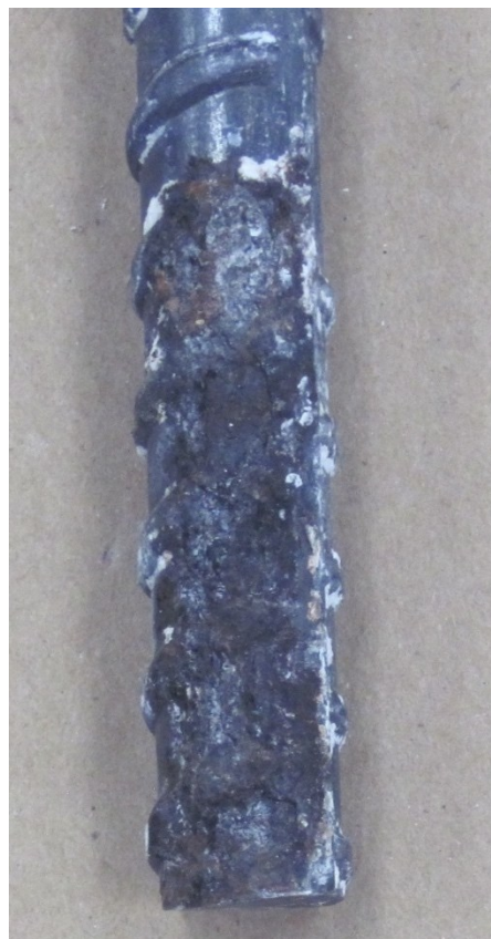
Figure 8-31. Corrosion spots observed on rebar 2 of sample STD3-MMFX-B.
