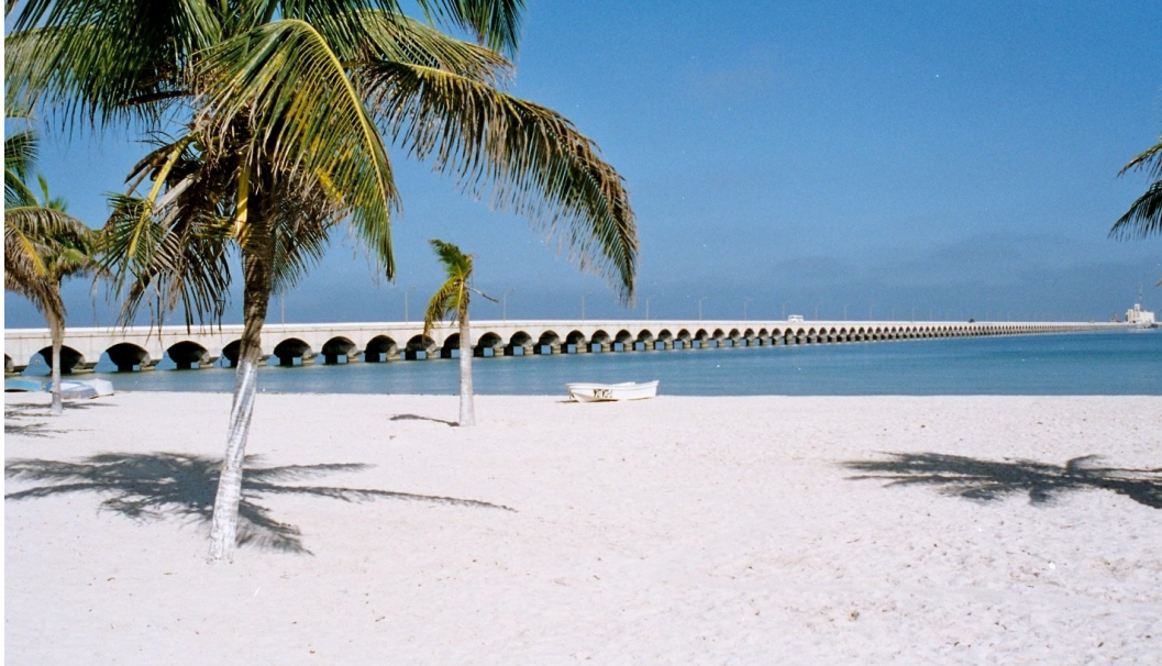
Figure 1-1. Progreso Pier located in Yucatan, Mexico, built with 304 round bars.
