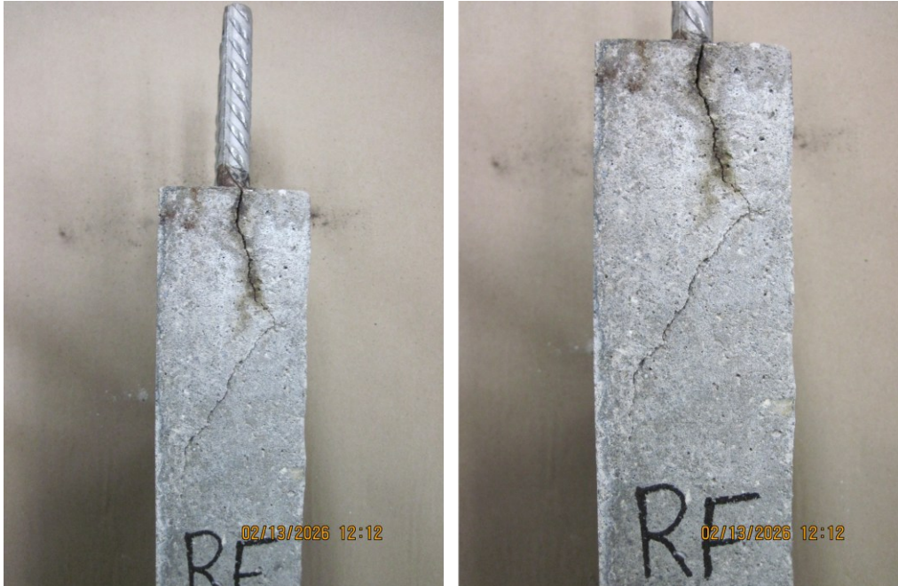
Figure 8-2. Right side crack of sample STD3-2101-B before termination.
