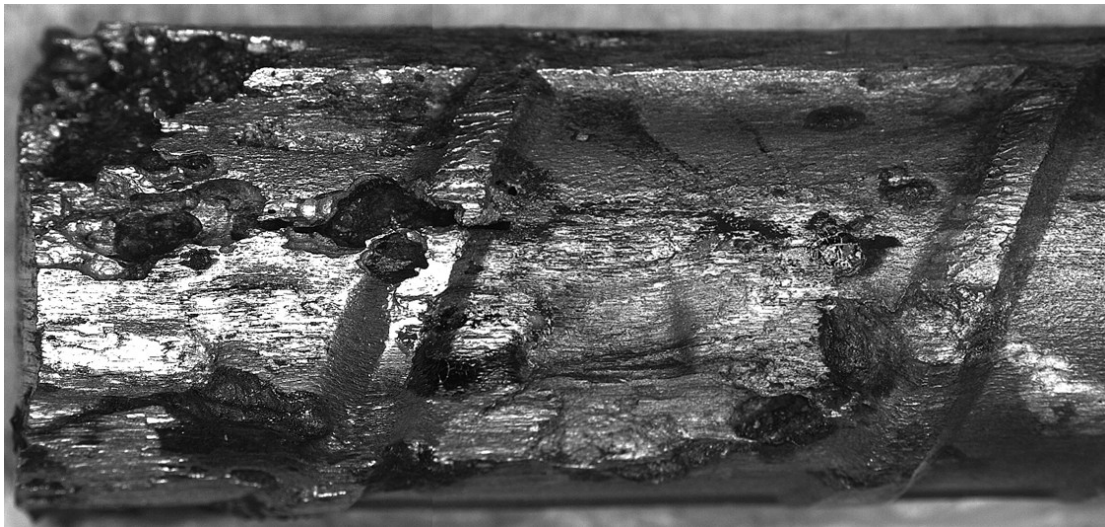
Figure 5-48. 2101 (Column A) rebar section close-up of the region with most corrosion.
