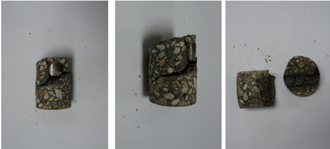
Figure 5-29. Images show the core obtained from column MMFX-1. It included a rebar segment.
