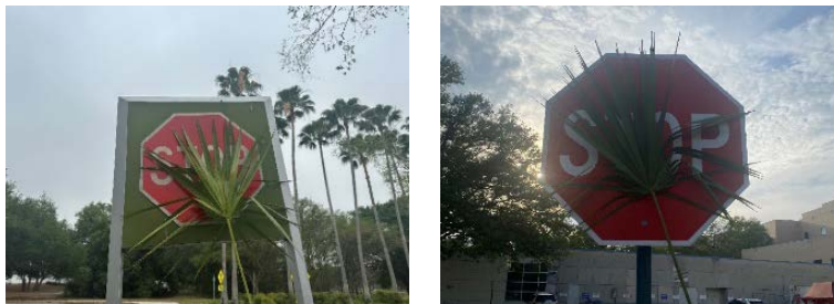
(c) Severe obstruction
