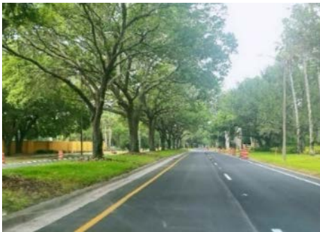
(a) Straight and clear lanes at daytime
