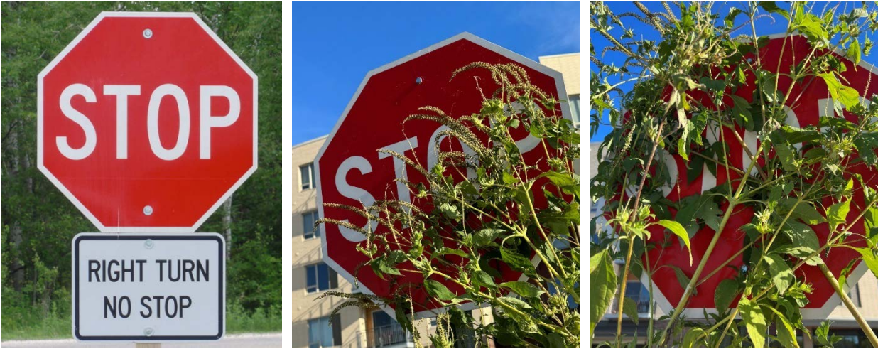
Figure 2-38 Illustration of different levels of obstruction on the stop signs.
