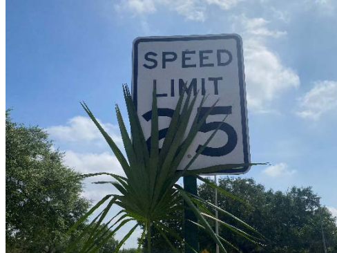
(d) Almost completely obstructing the number "2"
