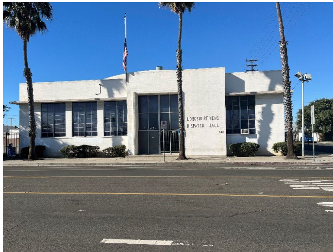
Figure 34. Longshoremen Dispatch Hall, Long Beach, California (Photo courtesy of author)
