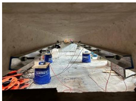
Skinny leg channel girder strengthened with aluminum channels
