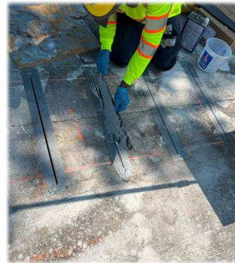
Installation of carbon fiber biscuits to improve lateral load distribution
