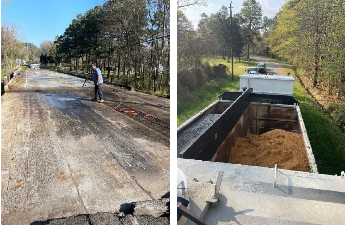
Figure 6.4 Pressure washing the surface and joints (left); LMC materials (right).
