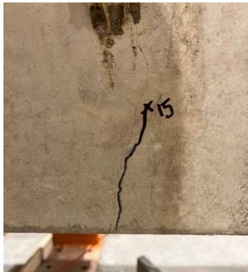
Figure 8.5 CL1: Flexural cracking at midspan after initial service level cycles.
