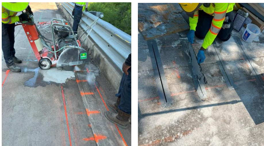
Figure 9.12 Cutting grooves (left) and installing biscuits (right).
