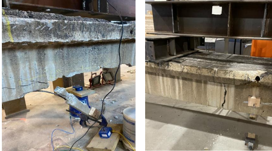
Figure 3.5 Flexural cracking and strand rupture near midspan.
