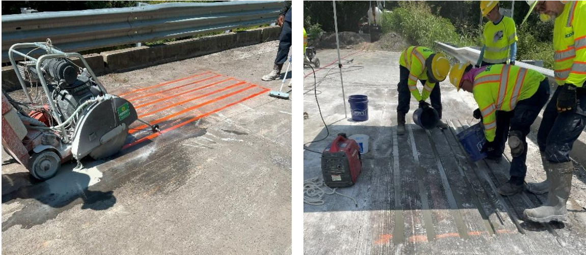
Figure 9.13 Cutting slots (left), NSM bar and grout installation (right).
