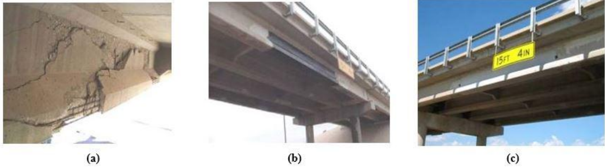
Figure 2.2 Bridge girder repair with externally bonded CFRP laminates: (a) impact-damaged beam; (b) continuous CFRP U-wrap after installation; (c) five years after repair (Yang et al. (2011)).
