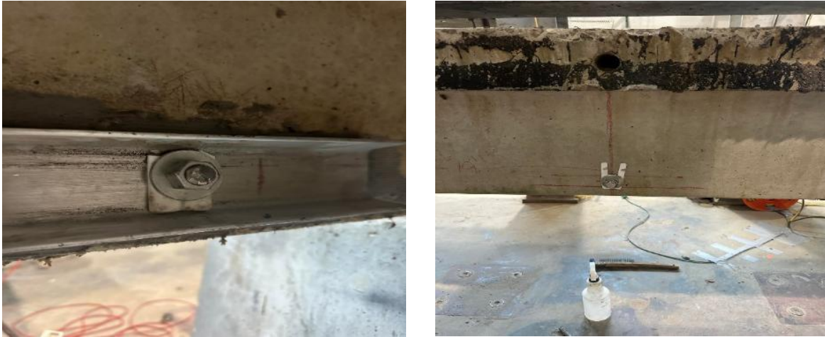
Figure 4.3 Aluminum channels bonded and through-bolted with aluminum threaded rods.
