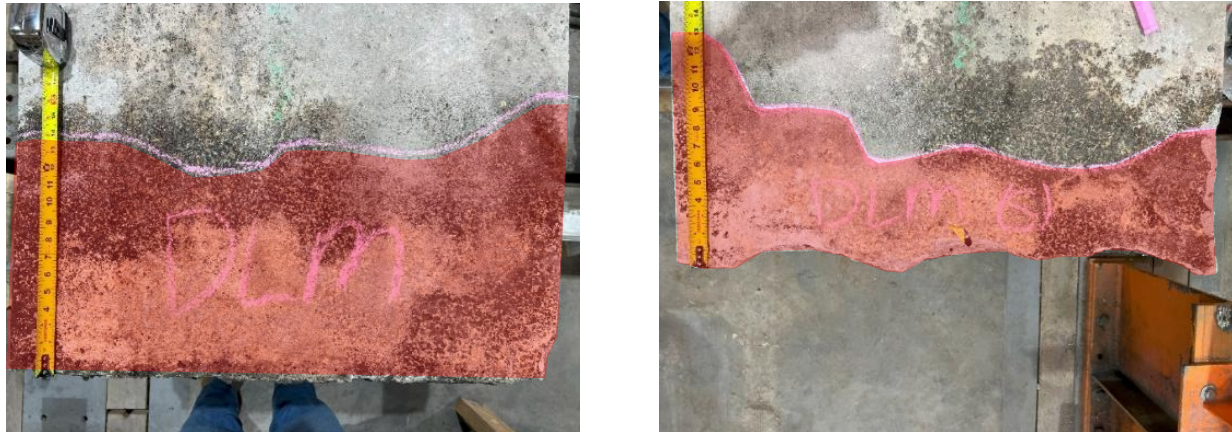
Figure 8.3 CL1 LMC delamination (highlighted in red) at north end (left); and south end (right).
