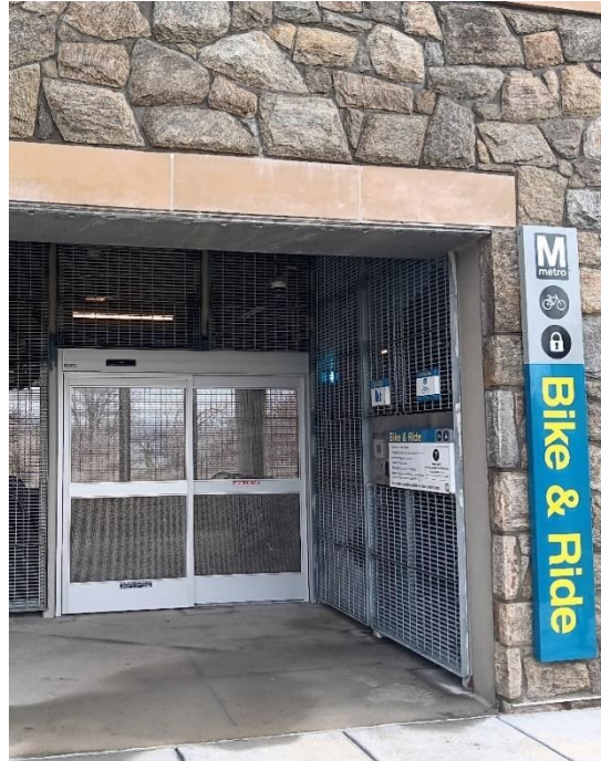
Photo 2. Bike storage room in Potomac Yard station on the Washington Metro.
