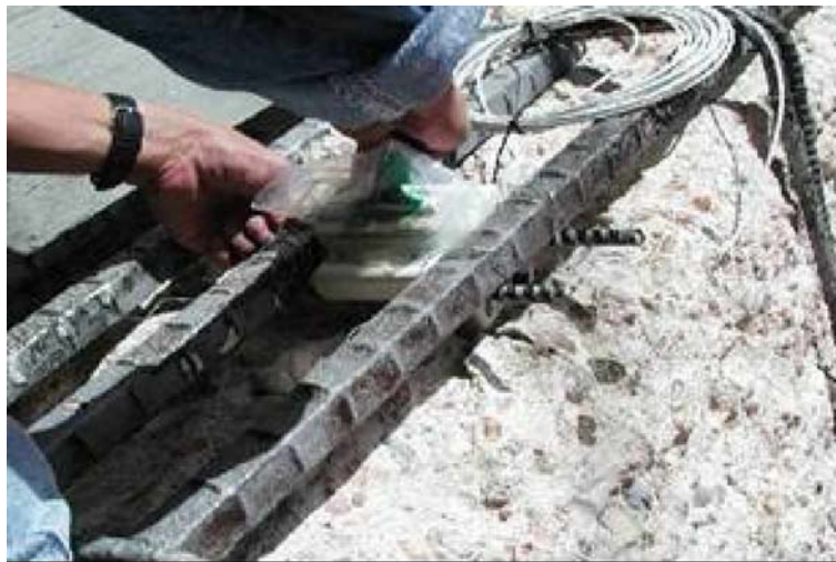
Figure 3-9 Installation of corrosion sensors during construction
