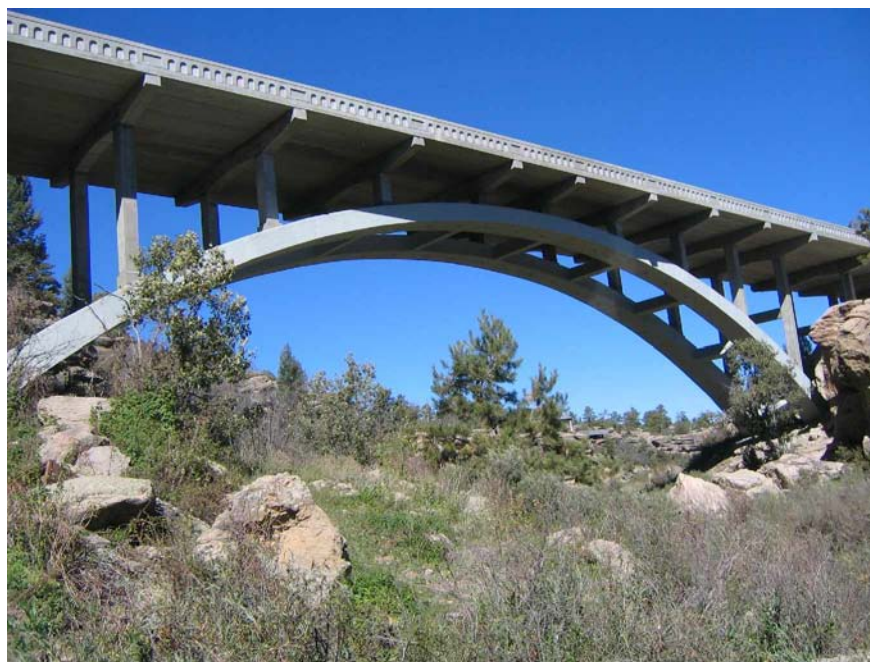
Figure 3-1 The repaired Castlewood Canyon Bridge
