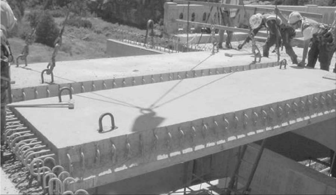
Figure 1-8 Precast deck panels
