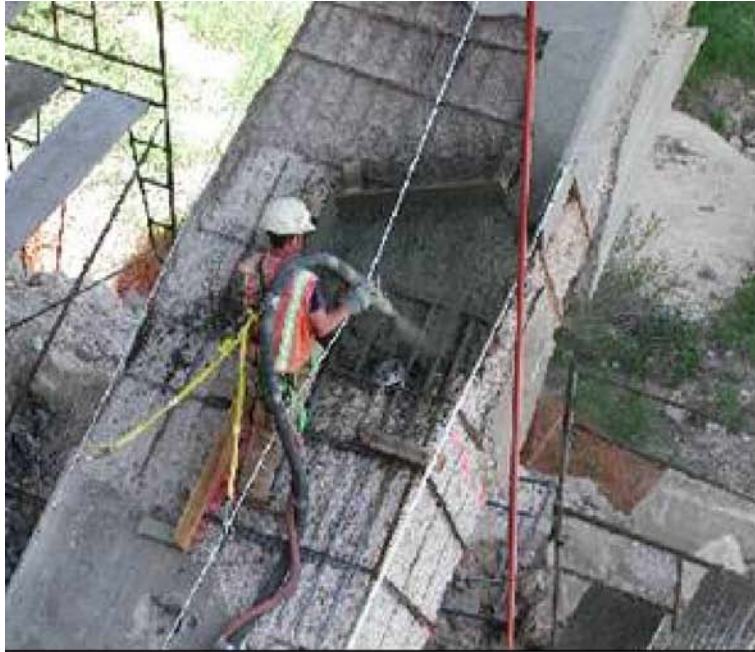
Figure 3-12 Shotcreting over corrosion instrument
