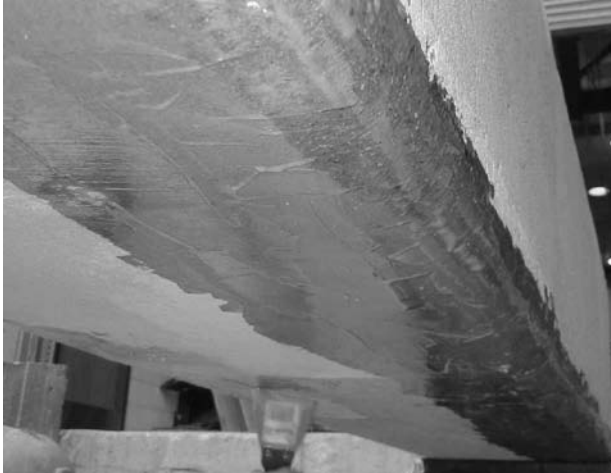
Step 1: Wetting surface with epoxy
