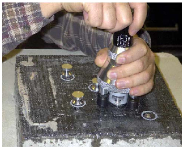
Figure 2-20 View of pull-off testing in progress
