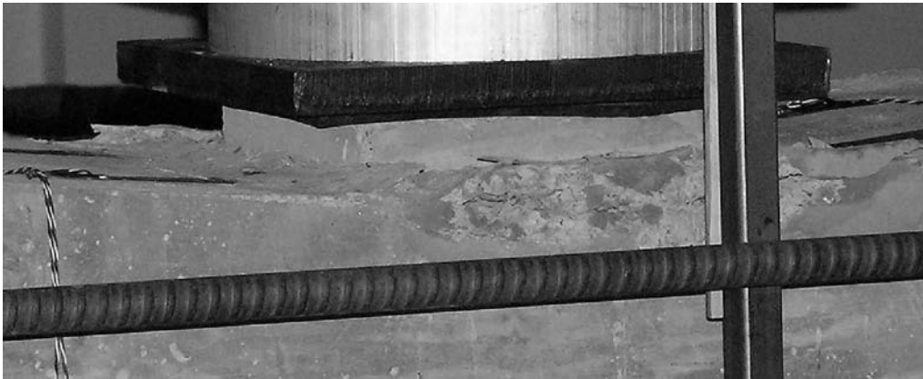
Figure 1-47 Concrete spalling around central cap (AC specimen)
