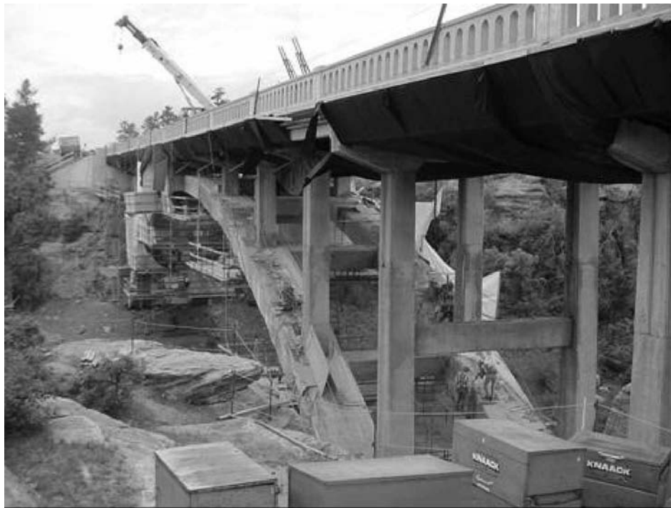
Figure 1-5 Arches during construction
