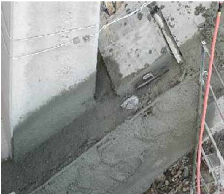
Figure 3-13 The embedded corrosion instrument (ECI-1)
