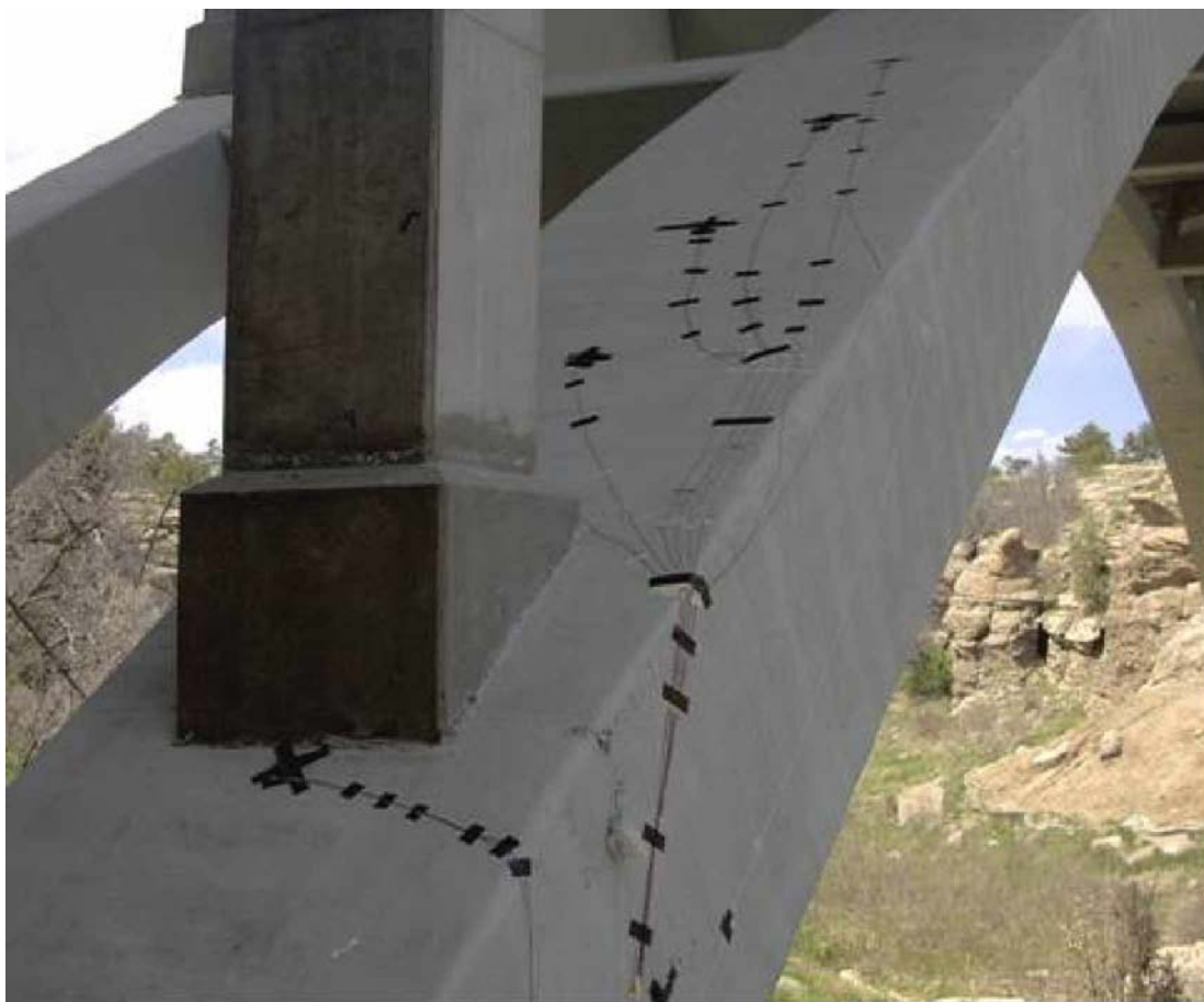
Figure 3-7 Wiring of strain gages - Extrados (Back)
