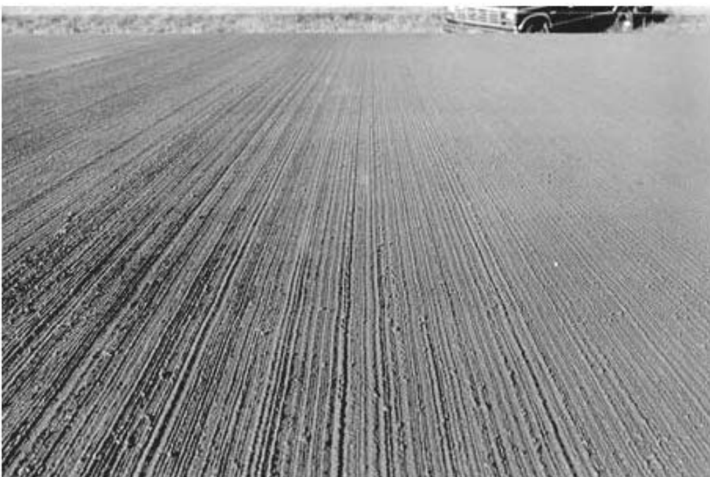
Photo 9: Close-up of transverse astro-turf texture
