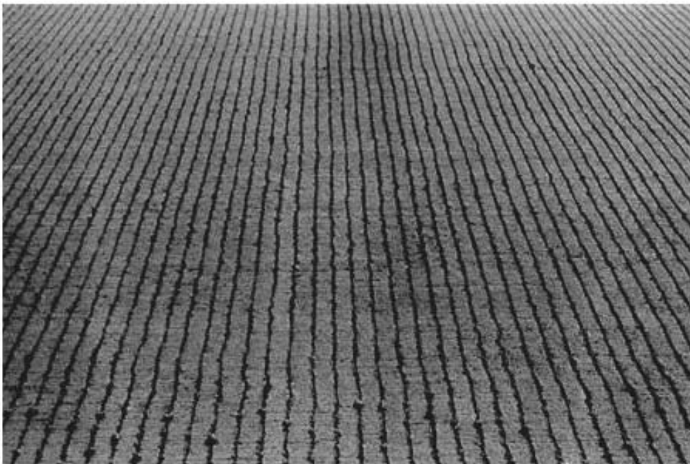
Photo 11: 1-inch uniform spaced transverse tining (state standard)
