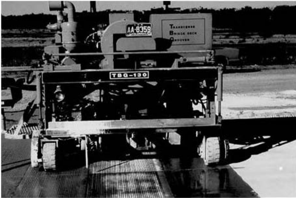
Photo 17: Installation of transverse grooves
