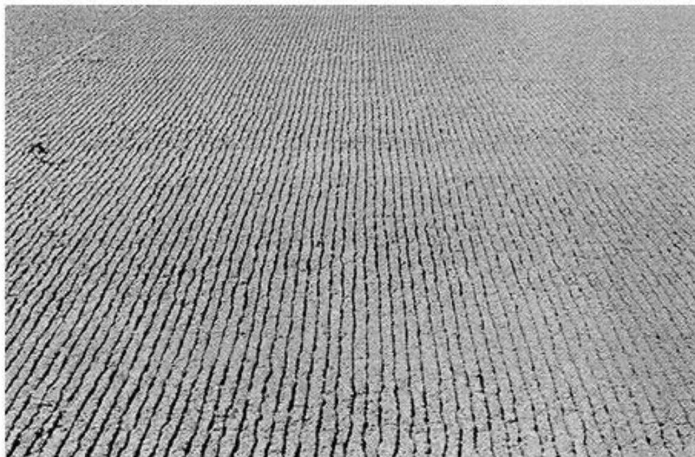
Photo 12: 1/2-inch uniform spaced transverse tining
