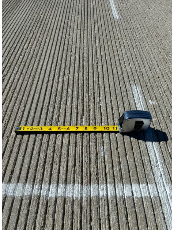
Figure 39. Photo. DGV section starting location.
