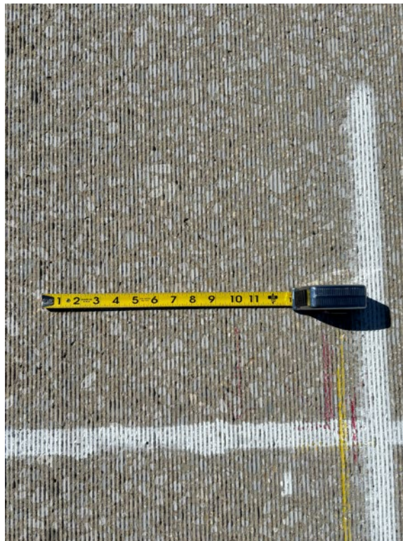
Figure 40. Photo. DGR section starting location.
