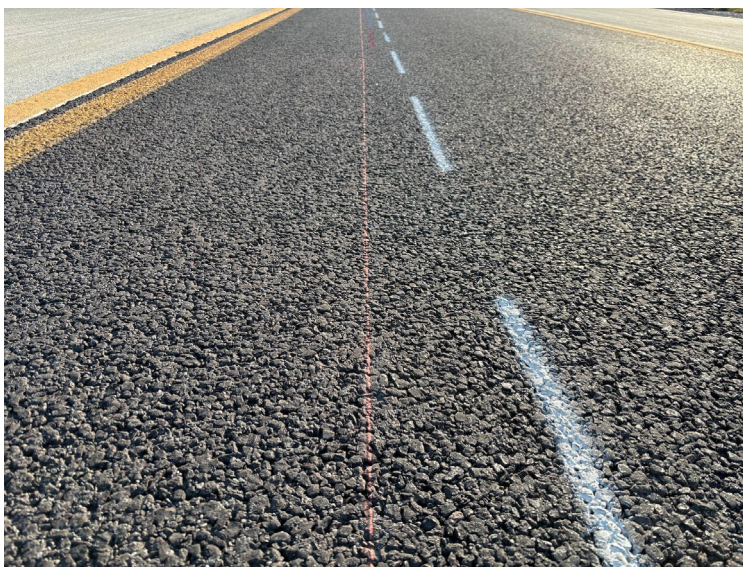
Figure 22. Photo. Chalk line placed to guide walking-speed profilers on the SMA section.
