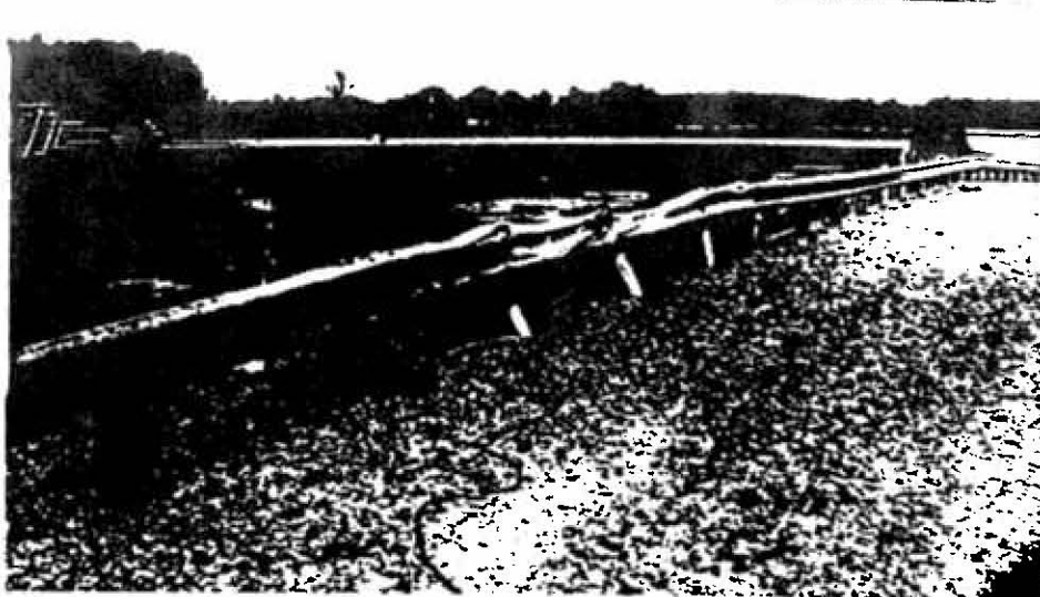
Figure 69. Post-test photographs of guardrail system, test 1862-9-90.
