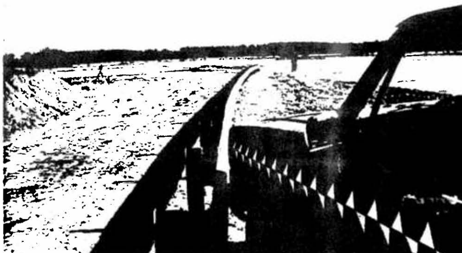
Figure 20. Pretest photographs of guardrail system, test 1862-3-89.
