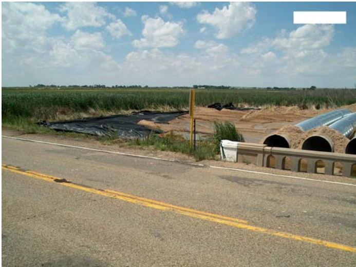
Figure 3.3 Use of geotextiles for the temporary protection of wetlands during construction of detour culverts on US Highway 50 by John Martin Reservoir in CDOT Region 2.
