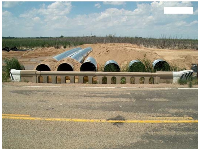
Figure 3.4. Construction of detour culverts within environmentally sensitive areas on US Highway 50 by John Martin Reservoir in CDOT Region 2.
