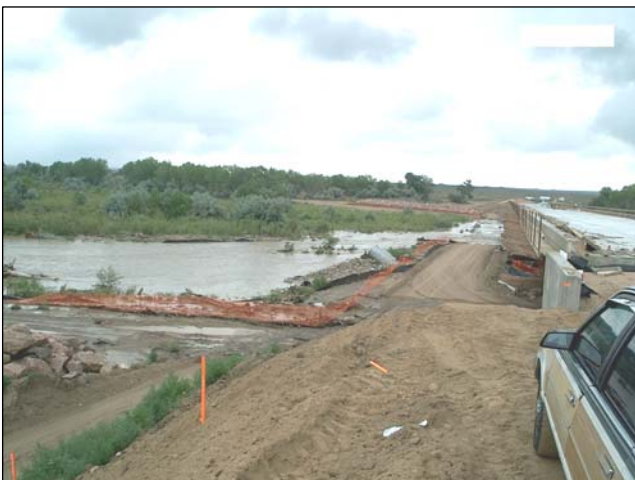
Figure 1.6. View of failed Pinon Bridge detour on Fountain Creek. Spring 2004 (CDOT Region 2).
