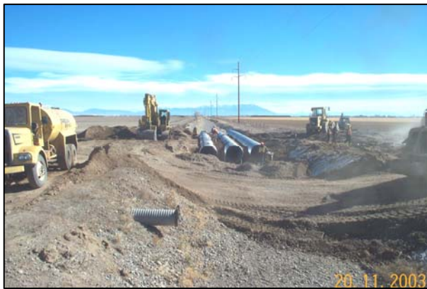
Figure 1.1 Construction of detour drainage structure. Three 60-inch pipes in Prairie Ditch under detour (CDOT Region 5).
