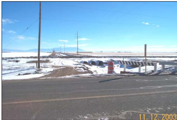
Figure 1.2. Construction of detour drainage structure. Three 60-inch pipes under Prairie Bridge detour (CDOT Region 5).
