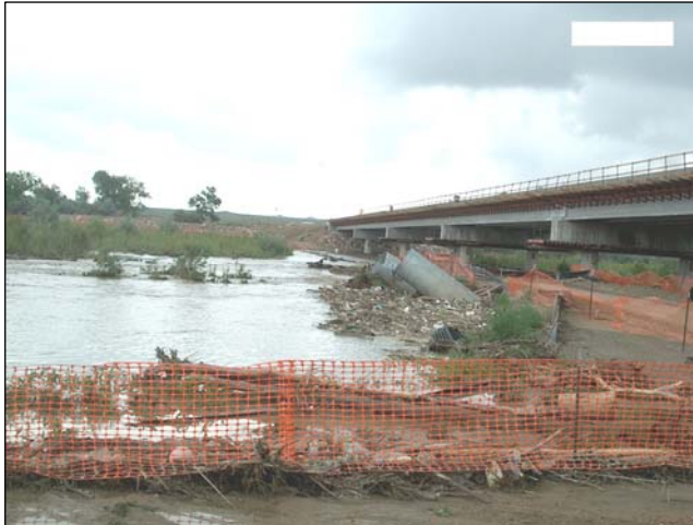
Figure 1.4. View of failed Pinon Bridge detour drainage structures on Fountain Creek. Spring 2004 (CDOT Region 2).
