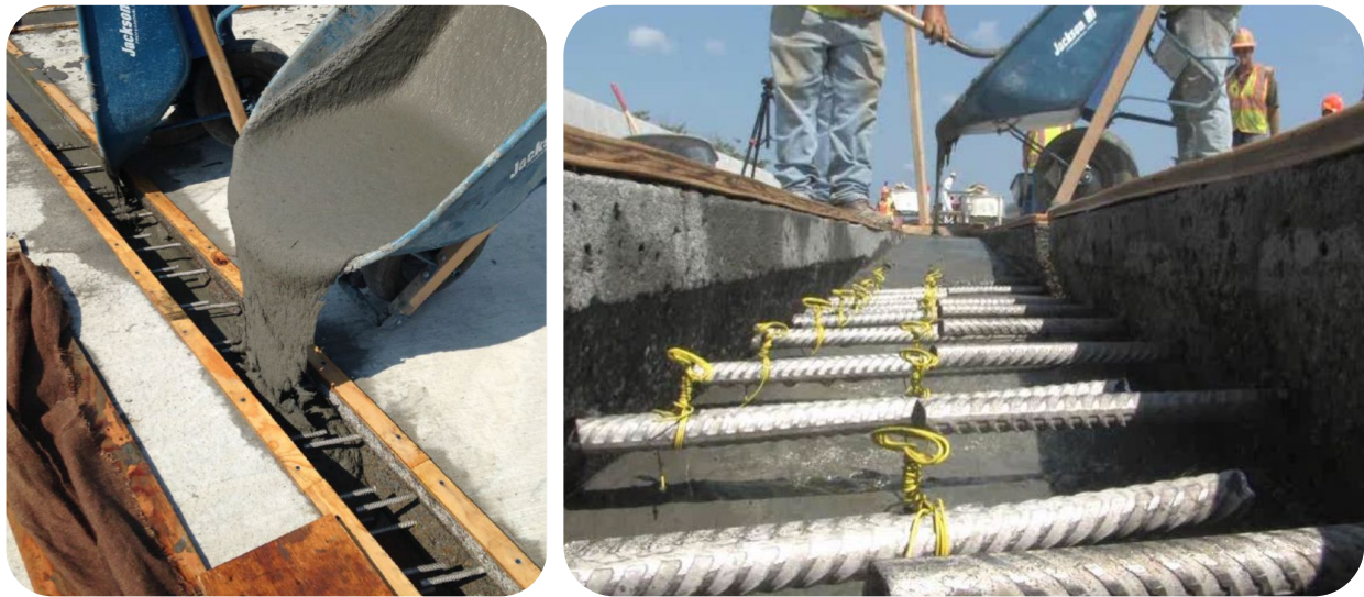
Figure 1-1: UHPC placement operation in a deck-level connection (Haber 2016)
