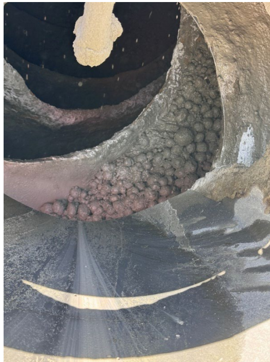
Figure 6-5: Cement Balls Present in the Mixture
