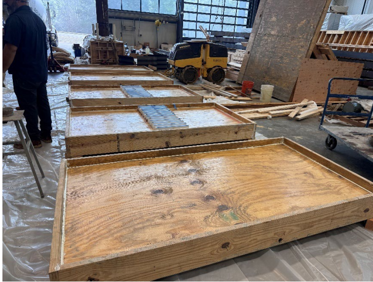
Figure 6-3: Formwork Constructed and Used in This Study
