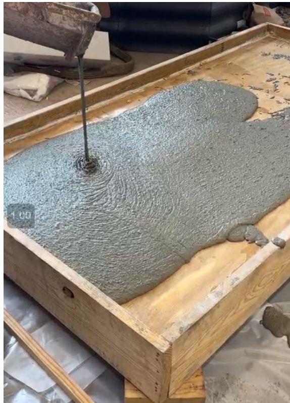
Figure 6-10: Placement of UHPC
