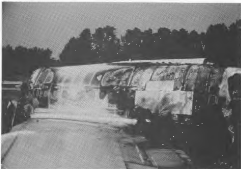
FIGURE 15. CV-880 PORT SIDE FIRE DAMAGE
