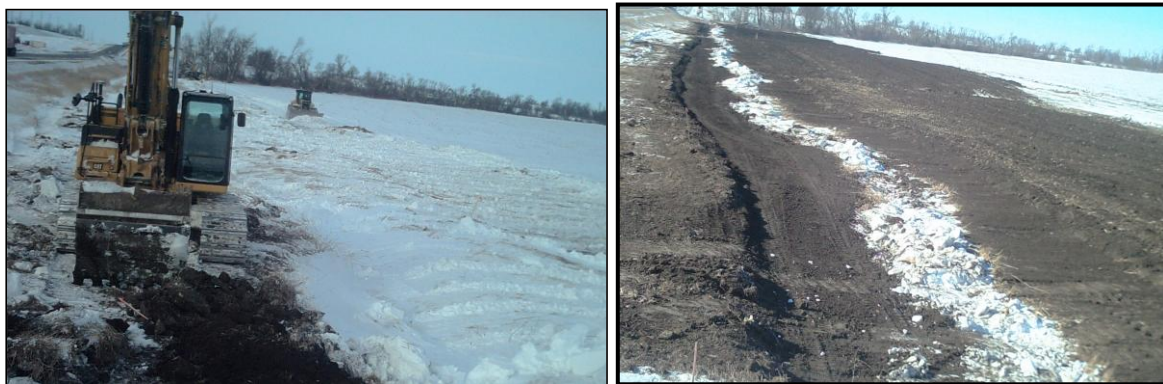
Figure 2-9. (Left) Excavation work initiated on January 17 and (Right) work finalized on January 21, 2022.
