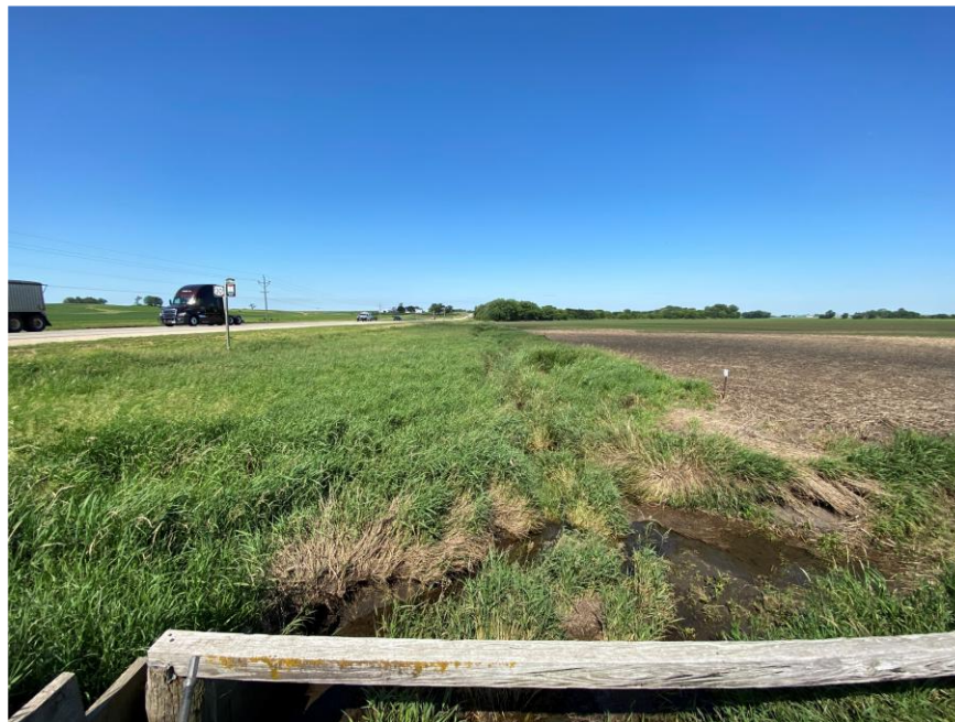
Figure 2-2. The roadside ditch prior to two-stage construction.
