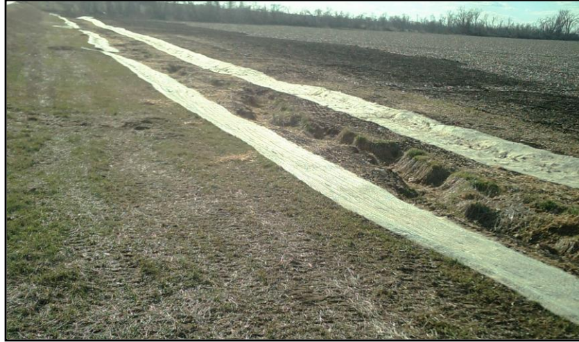
Figure 2-10. Seeding finalized at two-stage ditch site.
