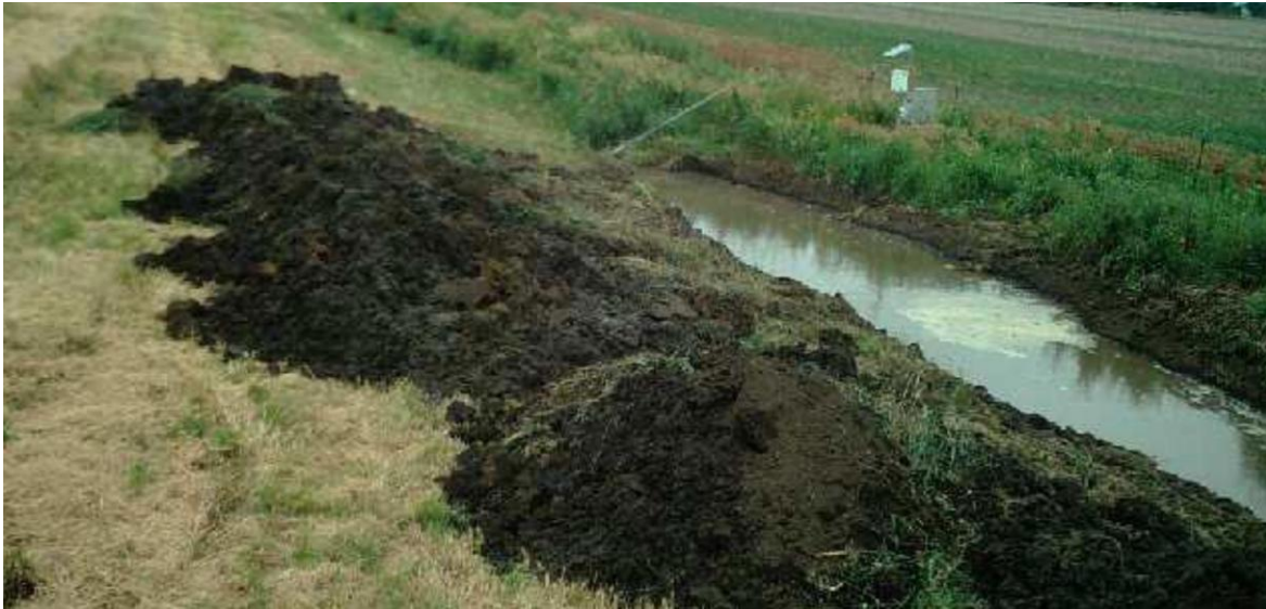
Figure 2-14. Excavation of the two-stage channel on June 19-22, 2024, that ended the monitoring project.
