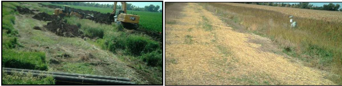
Figure 2-12. (left) Excavation of a portion of the ditch on June 13, 2023; (right) finished road grading and shoulder repair in close proximity of the ditch as seen on October 20, 2023.
