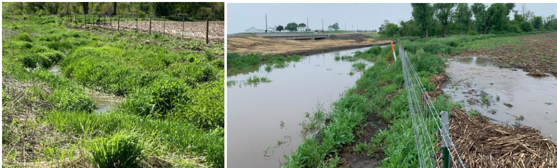
Figure 2-13. (left) Baseflow in the two-stage ditch on May 7, 2024. (right) Stormflow captured in the ditch on May 21, 2024.
