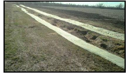
The finalized 2-stage ditch
