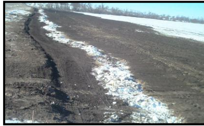
The 2-stage ditch under construction
