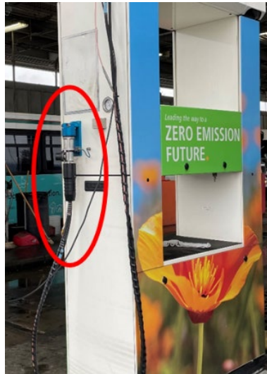
Figure 4. Example refueling receptacle for hydrogen buses
